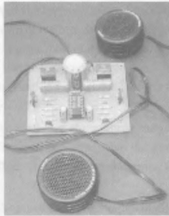
Figure 3.7.7 Panic generator mounted on a PCB
