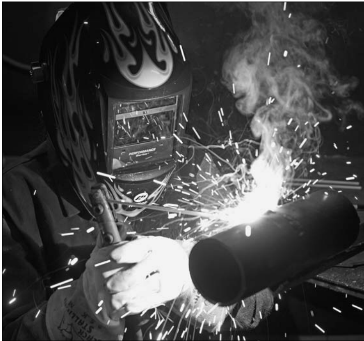
Figure 14-1: Steel pipe being stick welded.
