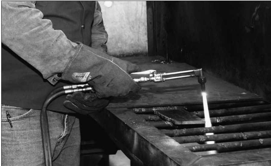
Figure 12-4: Operating an oxyfuel cutting torch.
