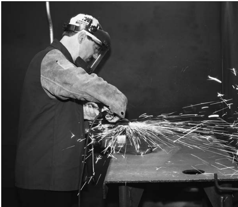
Figure 2-3: Cleaning steel with an angle grinder.
