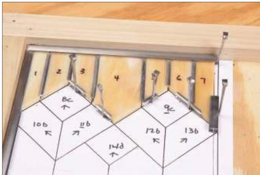
Figure 9-23: Using a \frac{3}{8} -inch lead gauge to help you trim the lead along the bottom of pieces 6 and 7.
