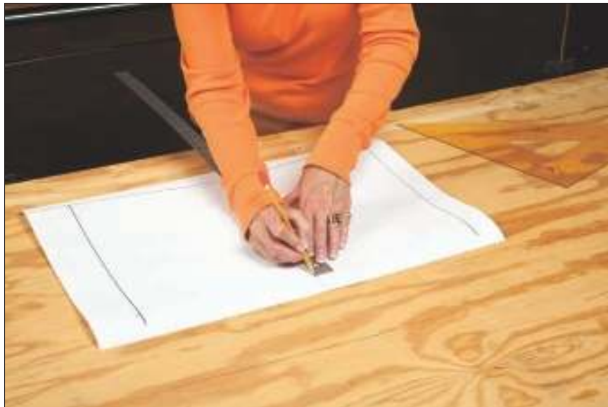
Figure 4-7: Marking the width of your panel using a ruler.
