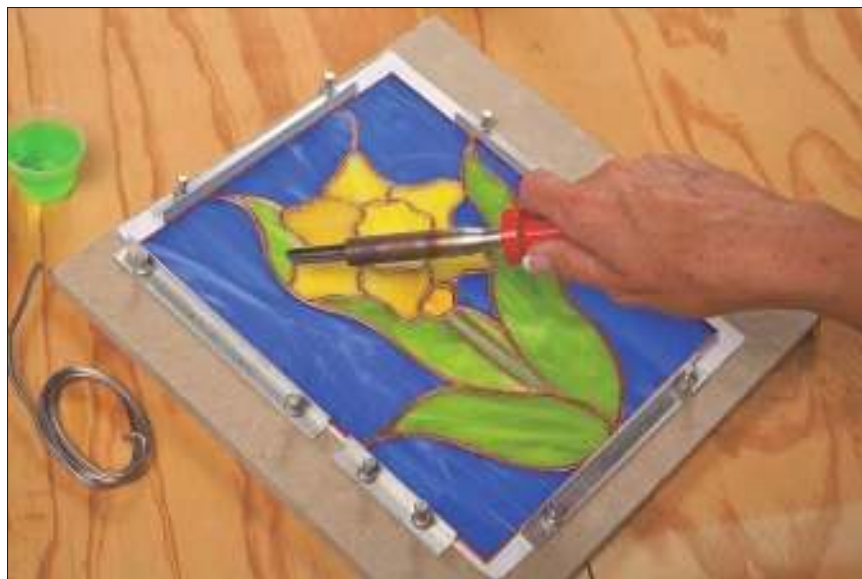
Figure 7-2: Holding your soldering iron the right way.
