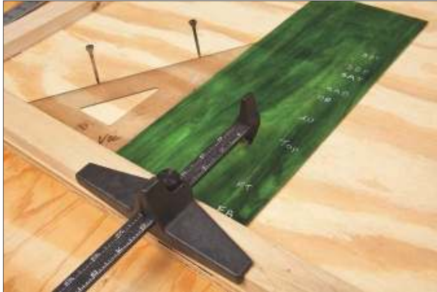
Figure 10-9: Glass set up and ready for stripping.
