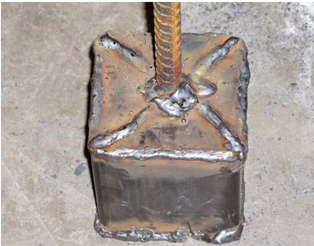
The can has been welded shut and a handle attached.
