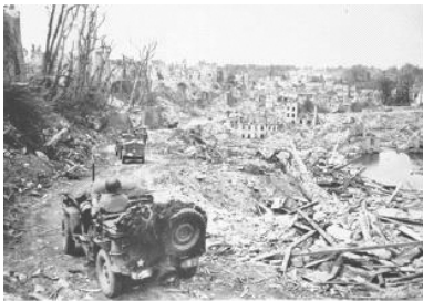
An American jeep snakes through the remains of Saint-Lô, which was obliterated during the assault of July 11-18, 1944. U.S. National Archives
