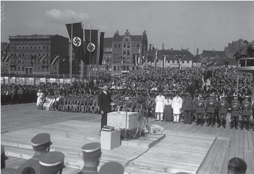
Schacht and the foundation stone for the new Reichsbank. May 5, 1934. Today the building is part of the Auswärtiges Amt, Germany's Foreign Office. Bundesarchiv.
