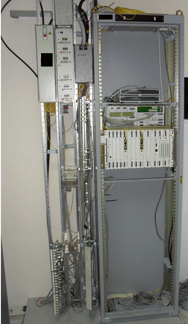
Fig. 3.2 Large size office demarcation point
