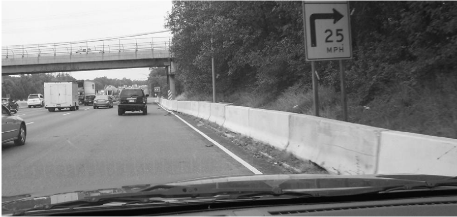
FIGURE 3.5 A Jersey Barrier [8]
