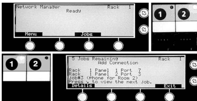
EXHIBIT 97.6 Intelligent patching. (Courtesy of SYSTIMAX Solutions; Richardson, TX.)
