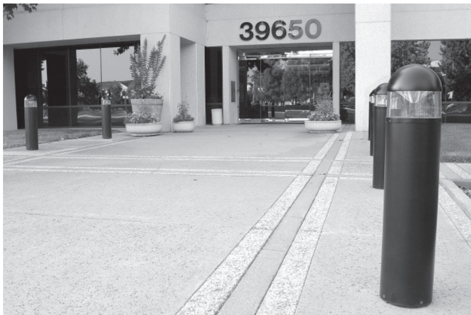
Figure 6-2 Sidewalks, lights, and landscaping can be used for protection.
