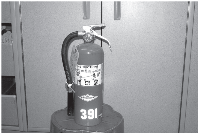
Figure 6-10 Portable extinguishers are marked to indicate what type of fire they should be used on.
