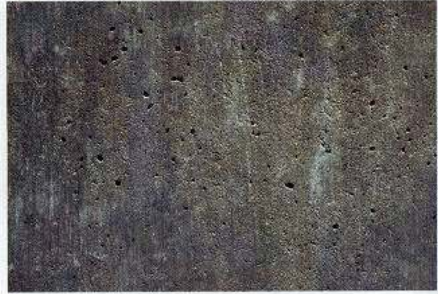
Concrete: Cast Concrete
