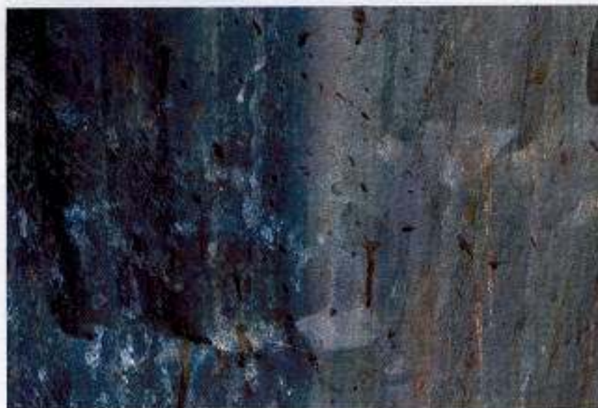
Metal Worn: Galvanized Steel
