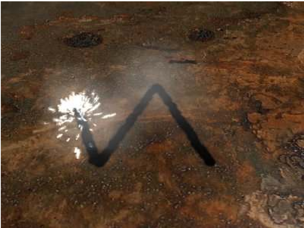
Figure 1101 Figure 8a: Sparks and Smoke
