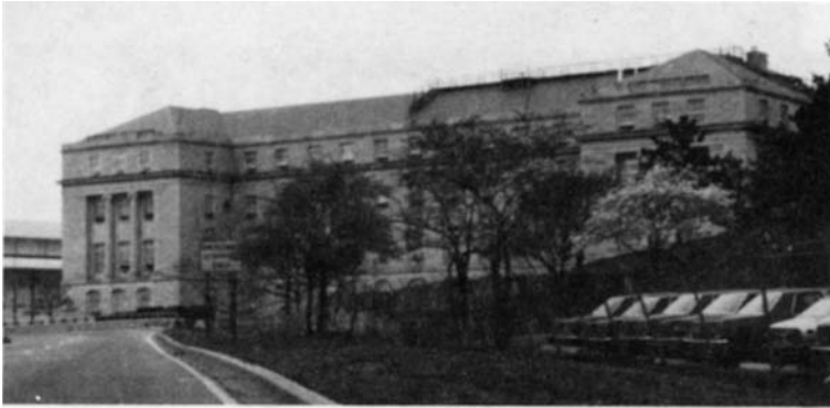
CIA's Technical Services Division (TSD) Building, where the research and development of E&E catalog items takes place.
