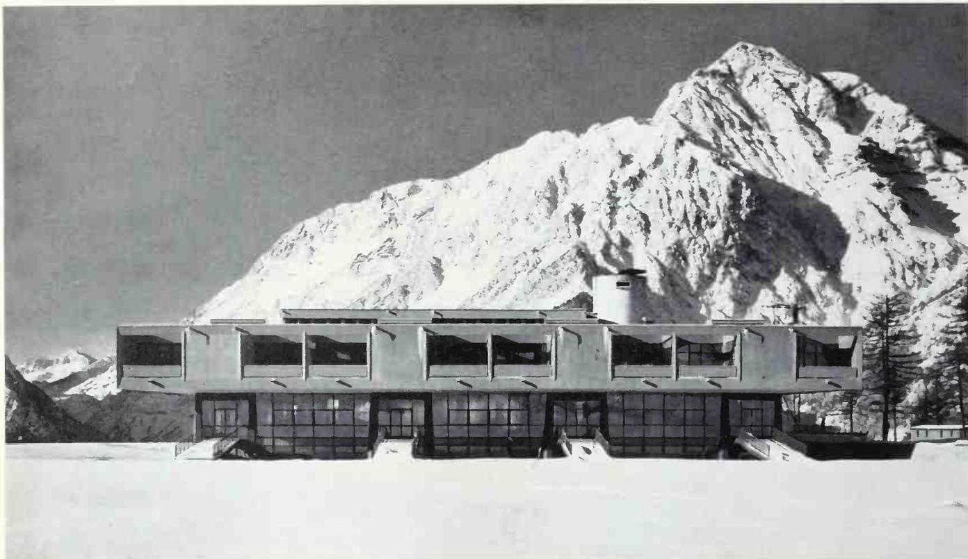
5. East side. In front of the top floor dormitories are roofless loggias. The roof of the penthouse, where the teaching staff are accommodated, can be glimpsed by the side of the staircase tower (cf. Fig. 1). Access is by bridges at main floor level.
