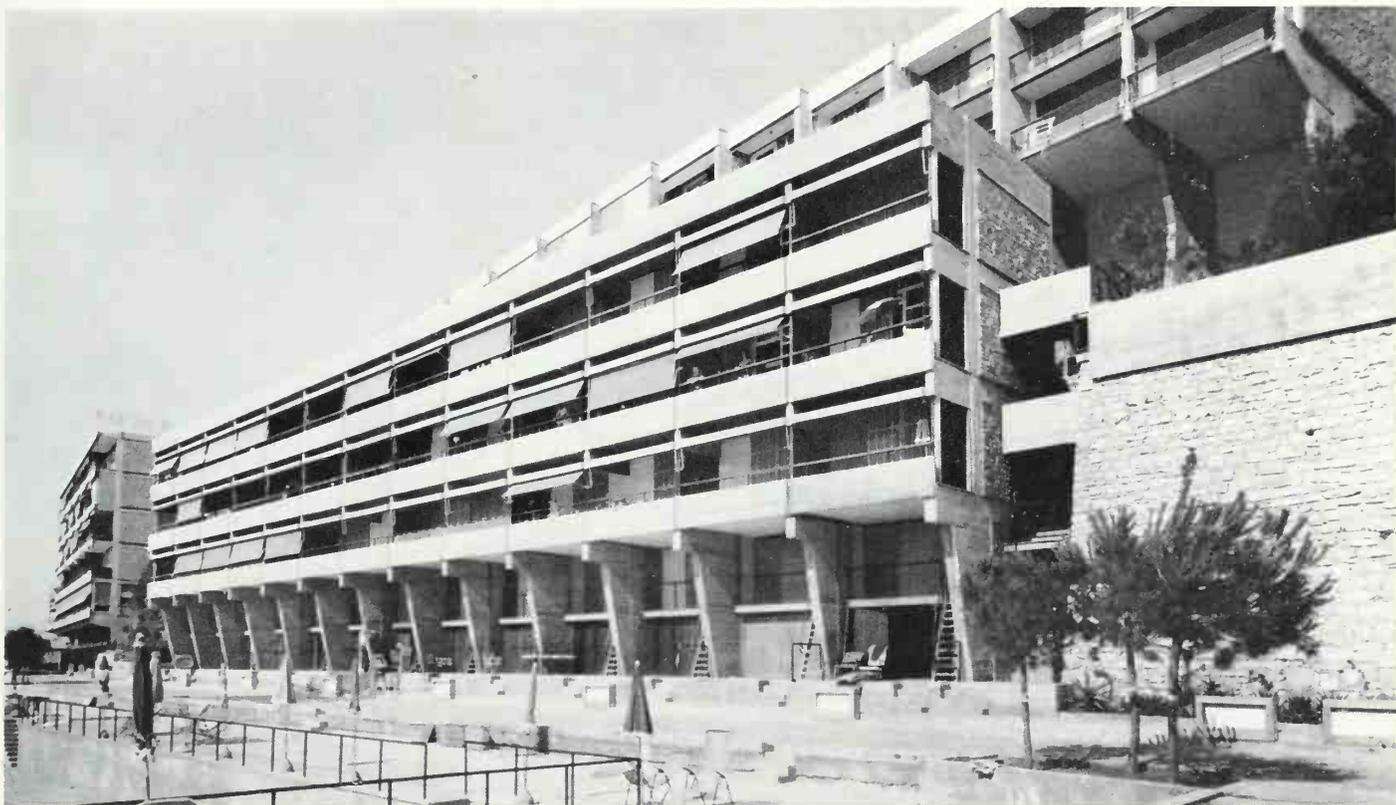
6. All the balconies can be sun-protected by awnings. The rough texture of the rubble walls is in attractive contrast to the exposed concrete faces.
