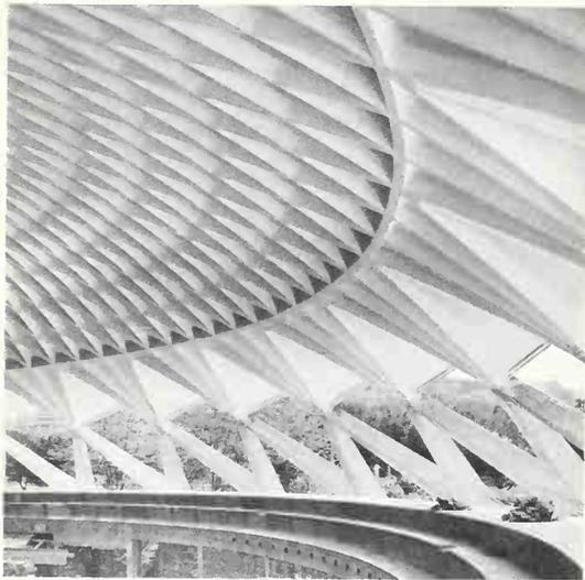
6. A close-up of the transition between roof shell and support.
