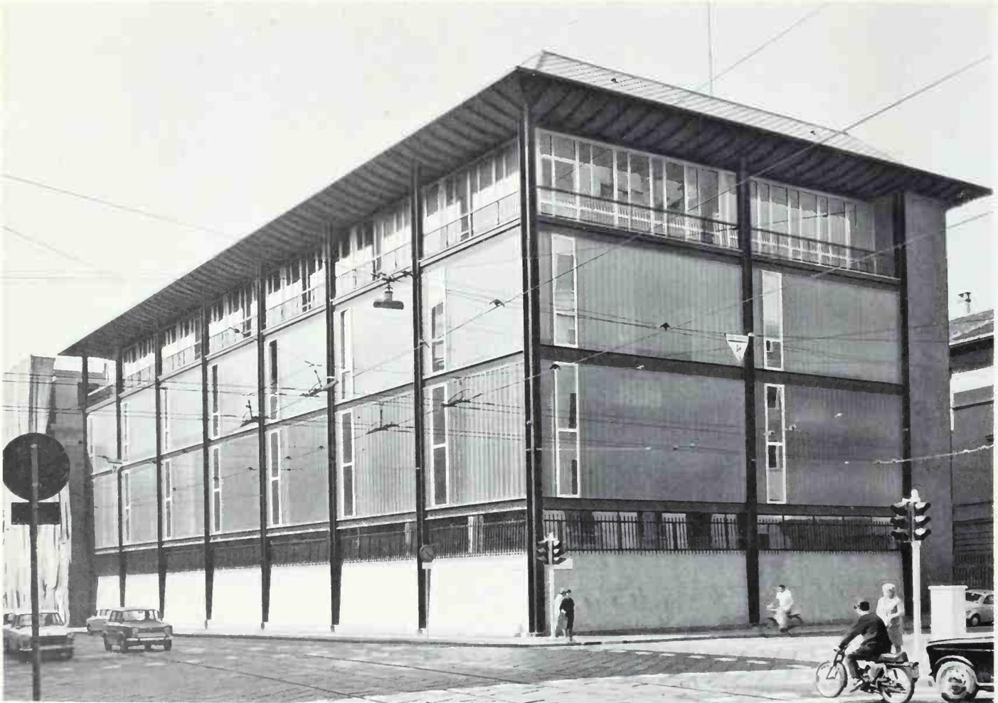
1. General view. The top light ribbon of the ground floor windows, which is repeated in enlarged form by the window ribbon of the top floor, is protected by crossbars.
