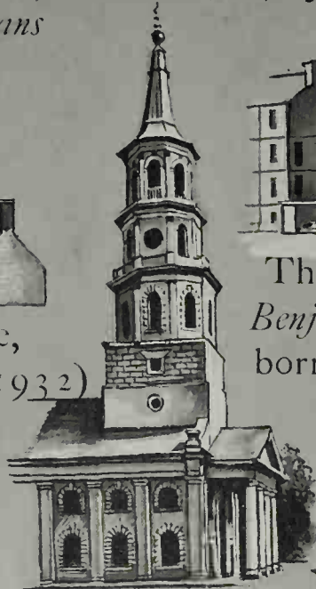
St Michael, Charleston, South Carolina, 1761
