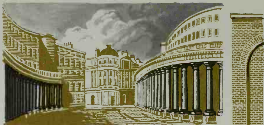
A The Quadrant, Regent Street 1818 Cast-iron columns
