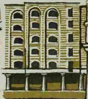
St Katherine's Dock, London, 1828: Telford
