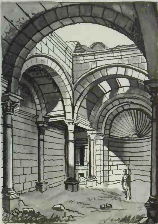
Cross-vault built of brick ribs and filled in with concrete Villa Sette Bassi, near Rome, c.A.D. 123-134
