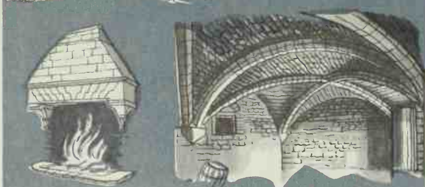
The Manor House, Boothby Pagnall, Lincolnshire, c.1180
