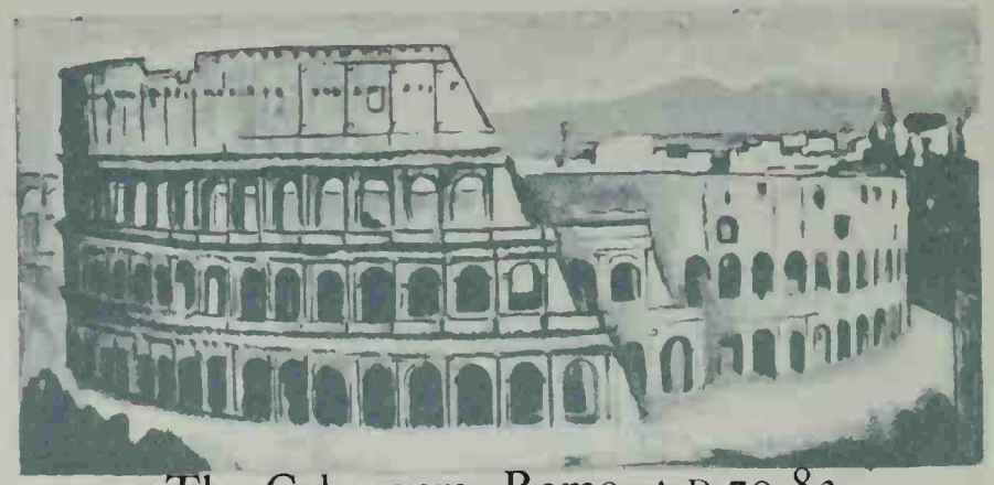
The Colosseum, Rome, A.D. 70-82 Designed for about 45,000 spectators. 80 piers support 3 tiers of arcading. Decorative use of superimposed orders of \frac{3}{4} external Doric, Ionic and Corinthian columns. Foundations: lava. Walls: brick and tufa. Vaults: pumice-stone. Facade: travertine blocks held by metal cramps. Columns and seats: marble
