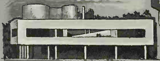
Villa Savoye, Poissy, nr. Paris, 1929-31. Reinforced concrete frame and piers, walls, brick & breeze blocks, floors and roof, hollow tiles.
