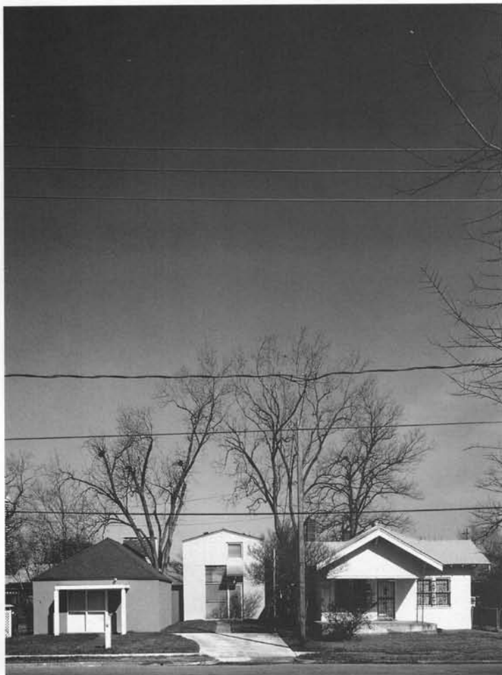
Main facade views
