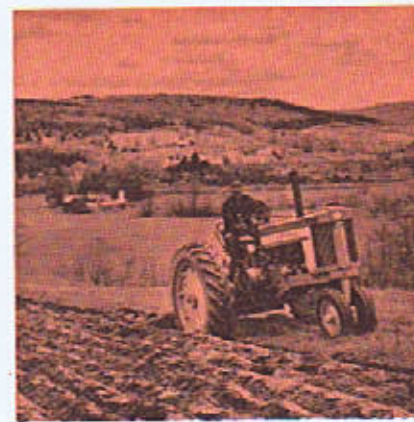
Halftone with tint plate: This is how a halftone appears when it is printed over a tint plate. It looks similar to a duograph.
