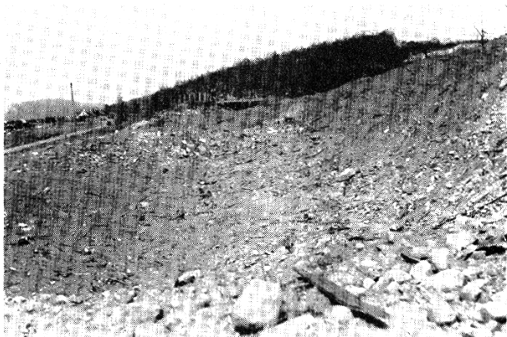
Lake Denmark Explosion. Site of building No. 9, the second to go.
