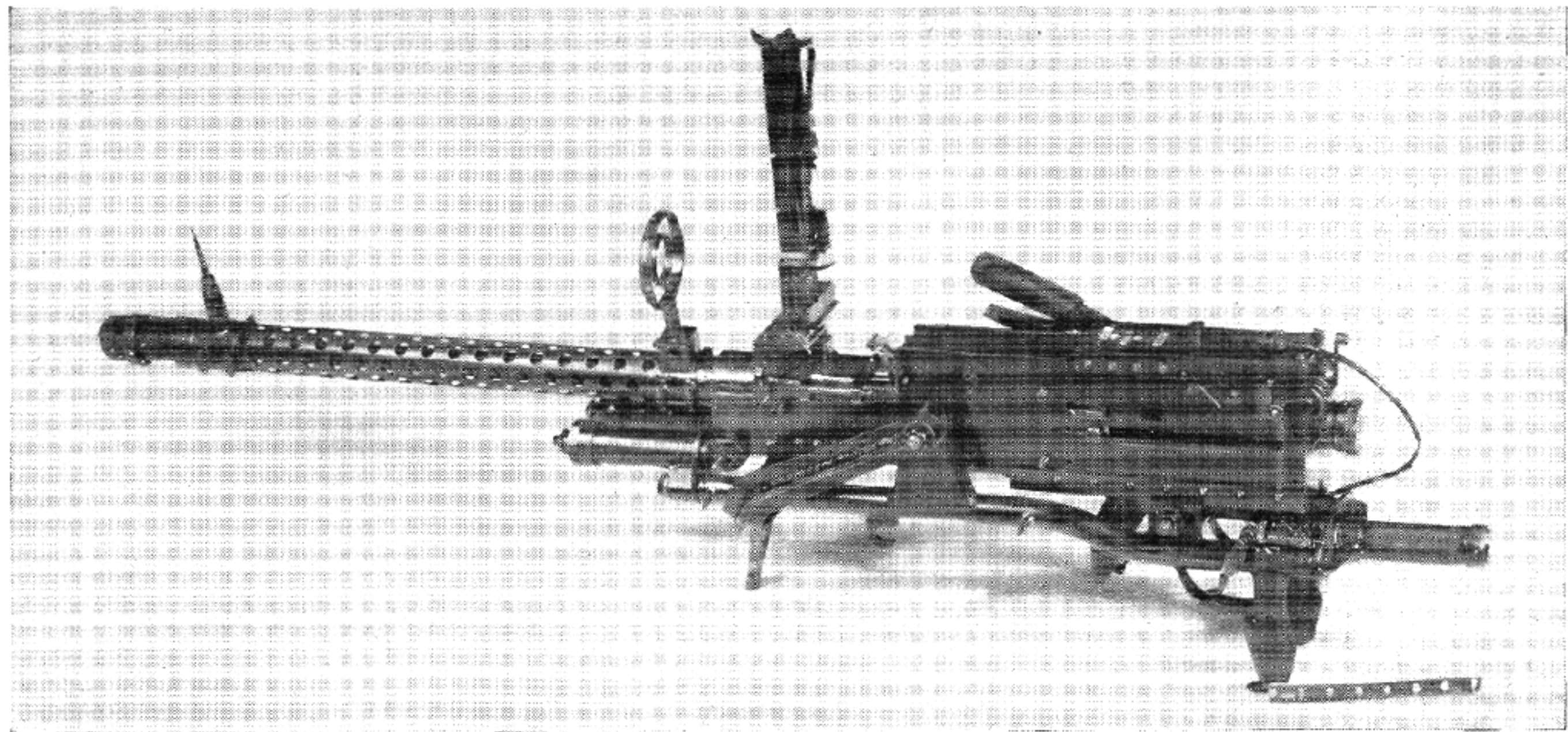
Japanese copy of Browning aircraft machine gun.
