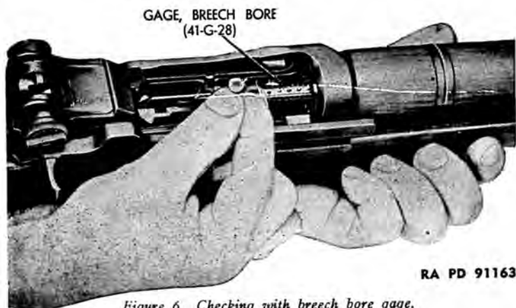
Figure 6. Checking with breech bore gage.
