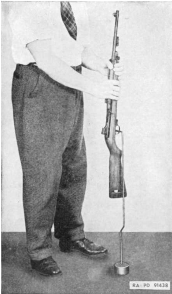
Figure 10. Testing Trigger pull.
