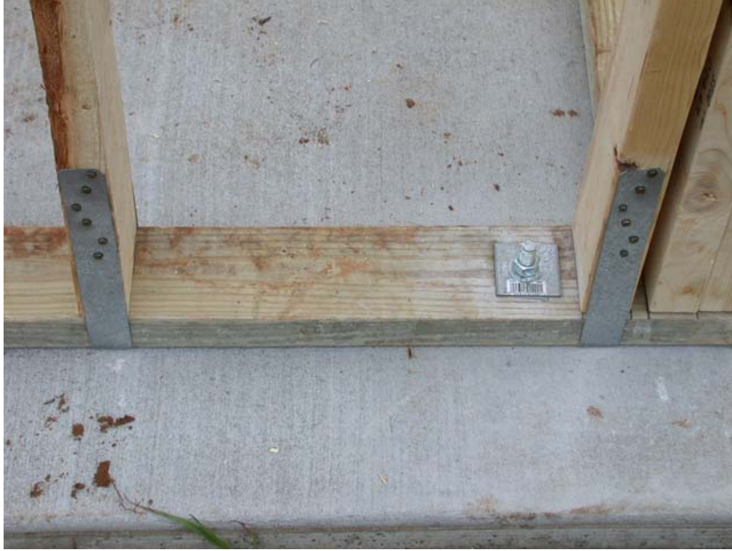
Bottom Plate Strap and Anchor Connection
