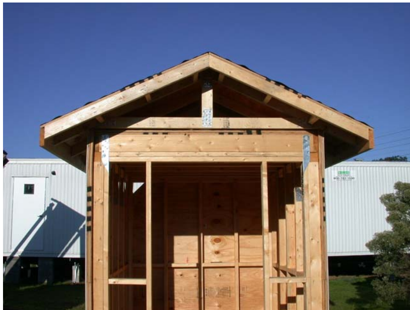
Gabled Roof Connection
