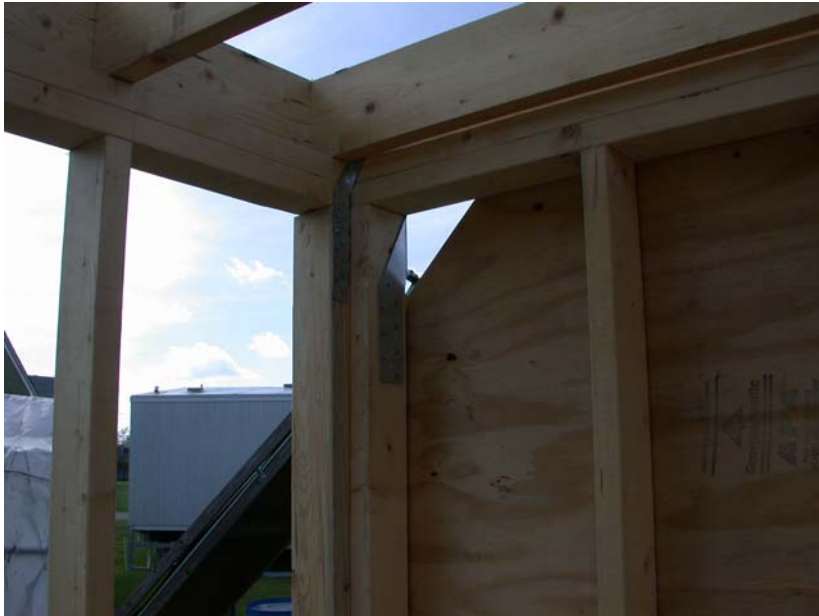
Roof-to-Wall Connection Detail
