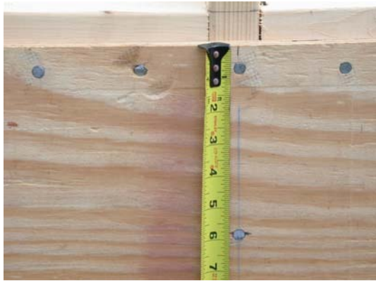
Plywood Attachment Spacing Detail
