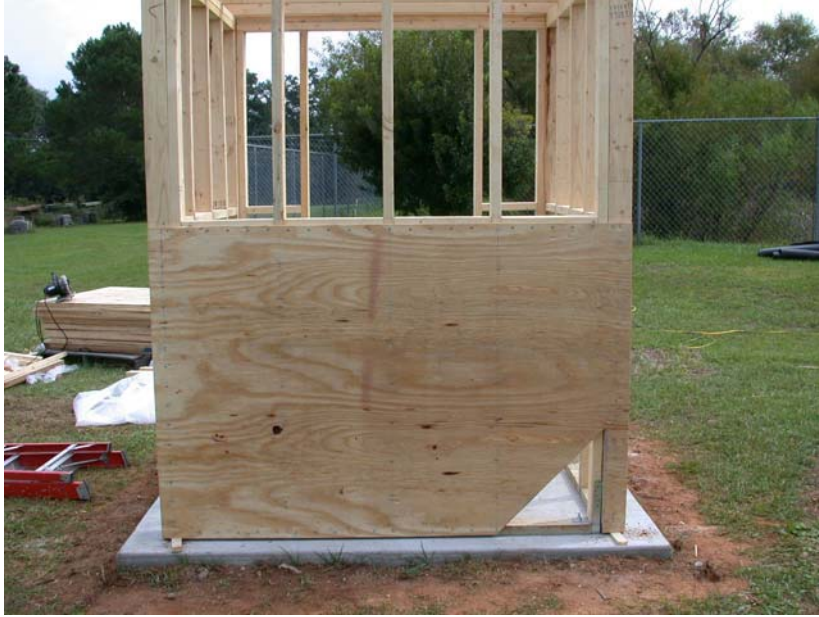
Plywood Sheathing Attachment
