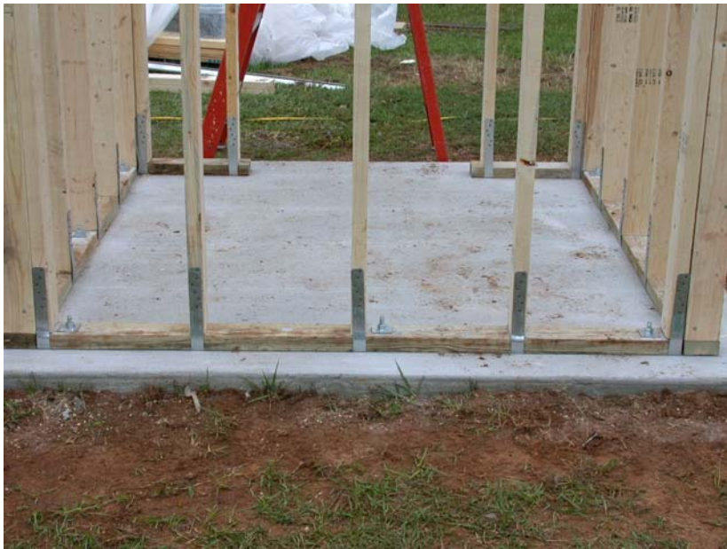
Anchor and Strap Detail
