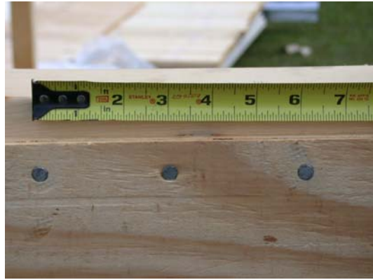
Plywood Attachment Spacing Detail
