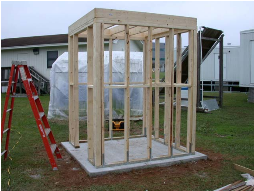
Stud Wall with Roof Joists
