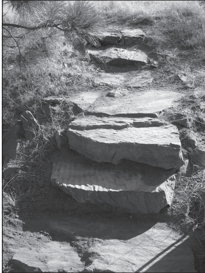
Figure 83—Each dry masonry rock step needs to contact the step below.
