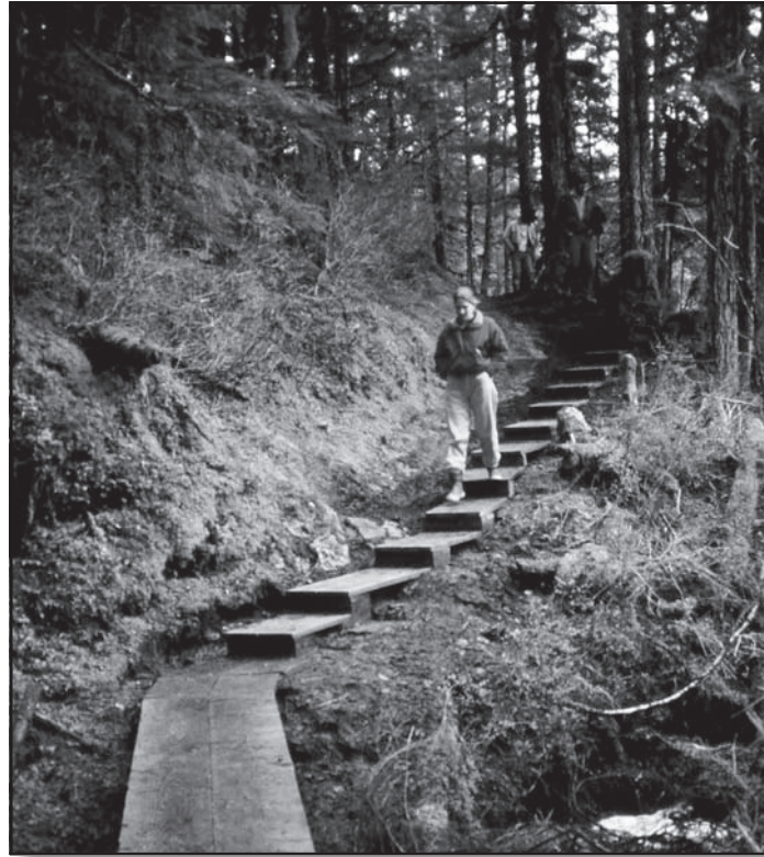
Figure 79—A step-and-run boardwalk in Alaska.
