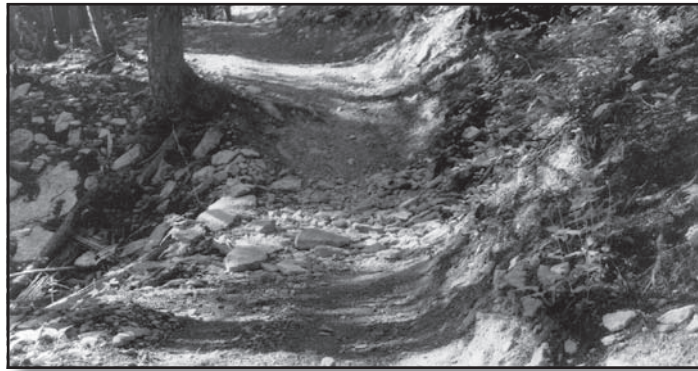
Figure 15—Rolling grade dips direct water off steeper sections on existing trails.
