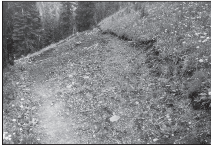
Figure 31—A classic case of tread creep. This trail needs help now because the tread is moving downhill.
