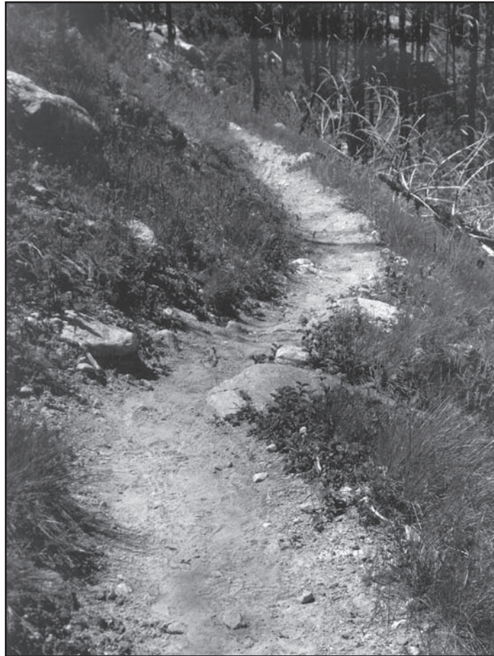
Figure 23—Rocks and logs help to keep the trail in place. Remember, this is a path through nature, not a monument to Attila the Hun.
