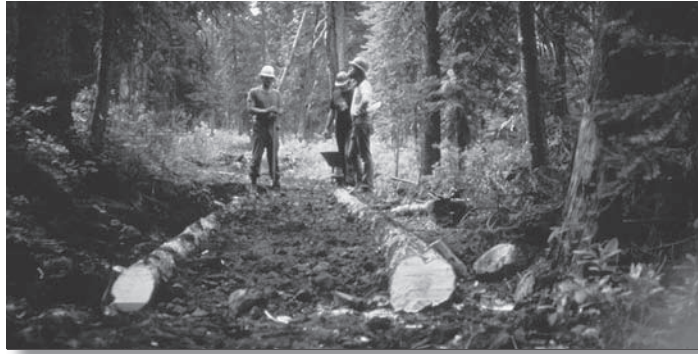
Figure 54—Subsurface puncheon covered with soil and rock.
