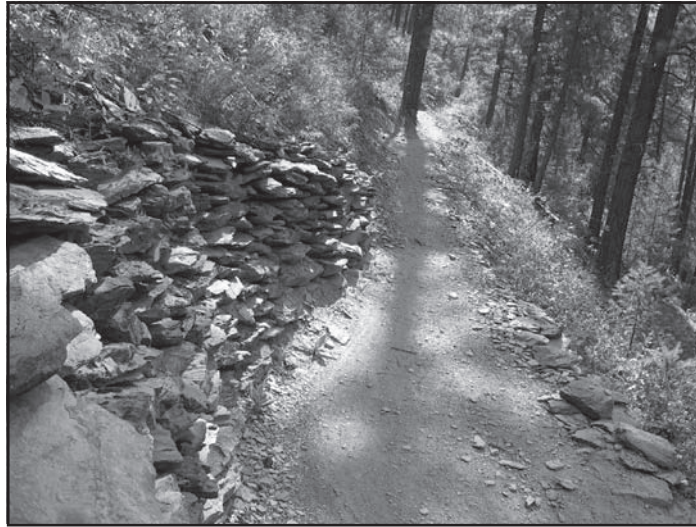
Figure 74—A rock retaining wall holding a steep, excavated backslope in place.
