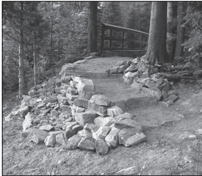
Figure 84—For stock use, landings should be long enough to hold all four of the animal's feet, or about 2 meters (6 ½ feet) long.
