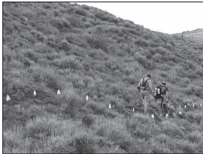
Figure 6—Pin flags mark the exact location of the trail tread and give you a good feel for the flow of the trail.
