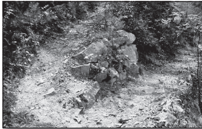
Figure 70—The rocks help prevent users from being tempted to cut this switchback.
