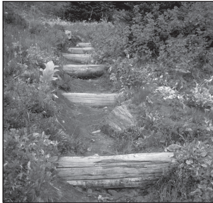
Figure 93—Over the years, this gully should fill in.
