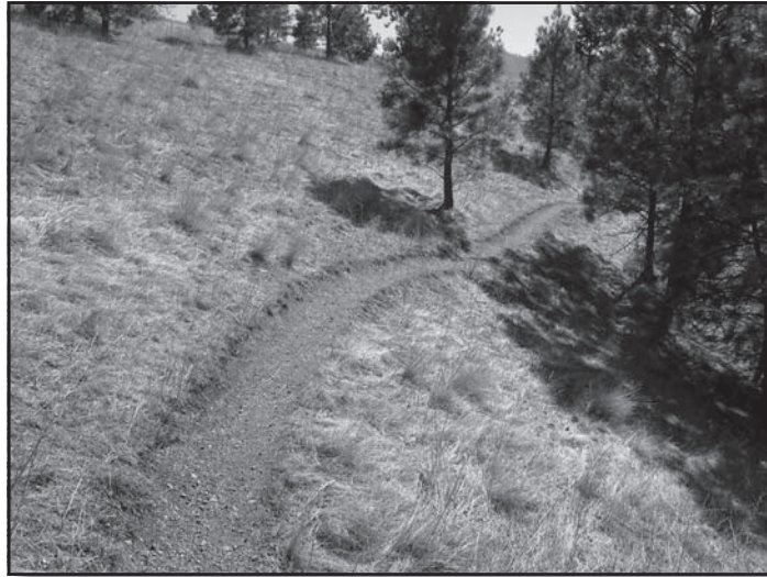
Figure 1—A rolling contour trail resists erosion.
