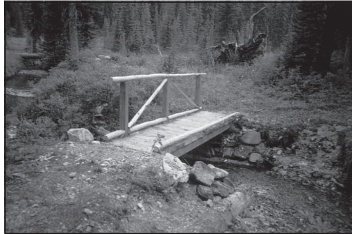
Figure 62—A simple footbridge with a handrail.
