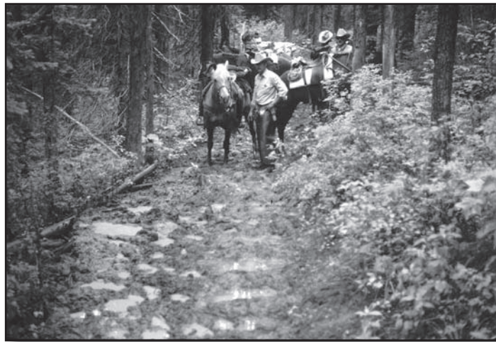
Figure 9—Standing water results in soft, boggy tread.
