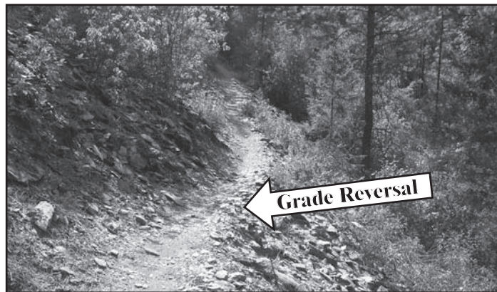
Figure 11—Grade reversals are much more effective than waterbars and require less maintenance. Grade reversals with outsloped tread are the drainage structure of choice.
