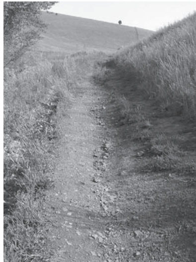
Figure 8—Water and gravity join forces to erode trail tread.
