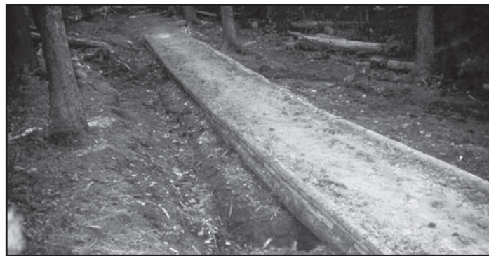
Figure 42—Turnpike maintenance includes recrowning the tread, cleaning out the ditches, and making sure the ditches are deep enough.
