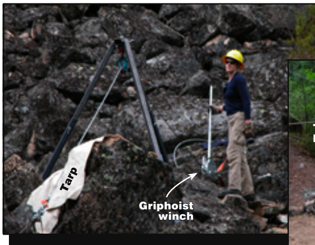
Figure 1—The portable tripod was used to move rocks downhill in this skyline operation with the load suspended from a cable. The operator used a Griphoist winch to control the cable tension. The tarp protects the cable from being damaged by the rocks.
