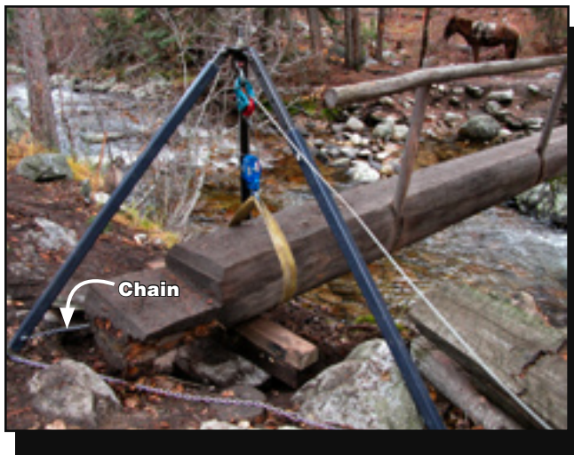
Figure 7—One portable tripod can be used by itself when lifting heavy objects, such as one end of a log bridge. The safety chain around the bottom prevents the legs from spreading too far apart. Hooks welded near the bottom of each leg hold the chain in place.
