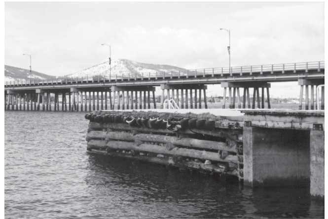
Figure 11—This aging crib dock continues to provide sturdy recreation access in a lake that is subject to icy conditions.
