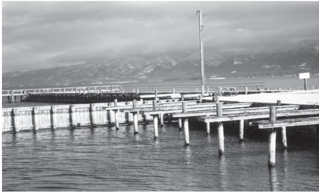
Figure 12—Small pile-based docks (finger docks) reaching out from the main dock offer access during periods of high water.
