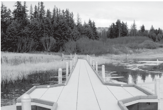
Figure 15—Side extensions to this floating trail bridge provide places where users can stop without obstructing others (photo by Paul Schrooten, USDI Fish and Wildlife Service).
