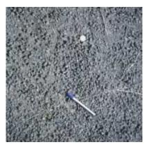
Figure 6. Macadam surface with blotter sand blown away.
