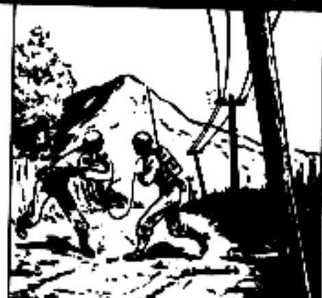
HIGH TENSION LINES
