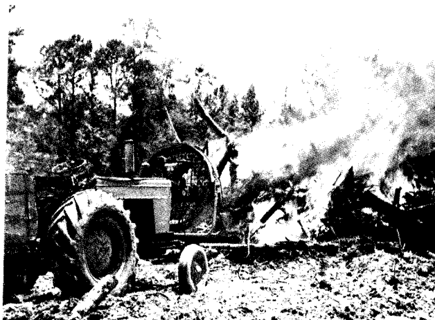
Figure 3-35. Heavy duty brush burner.
