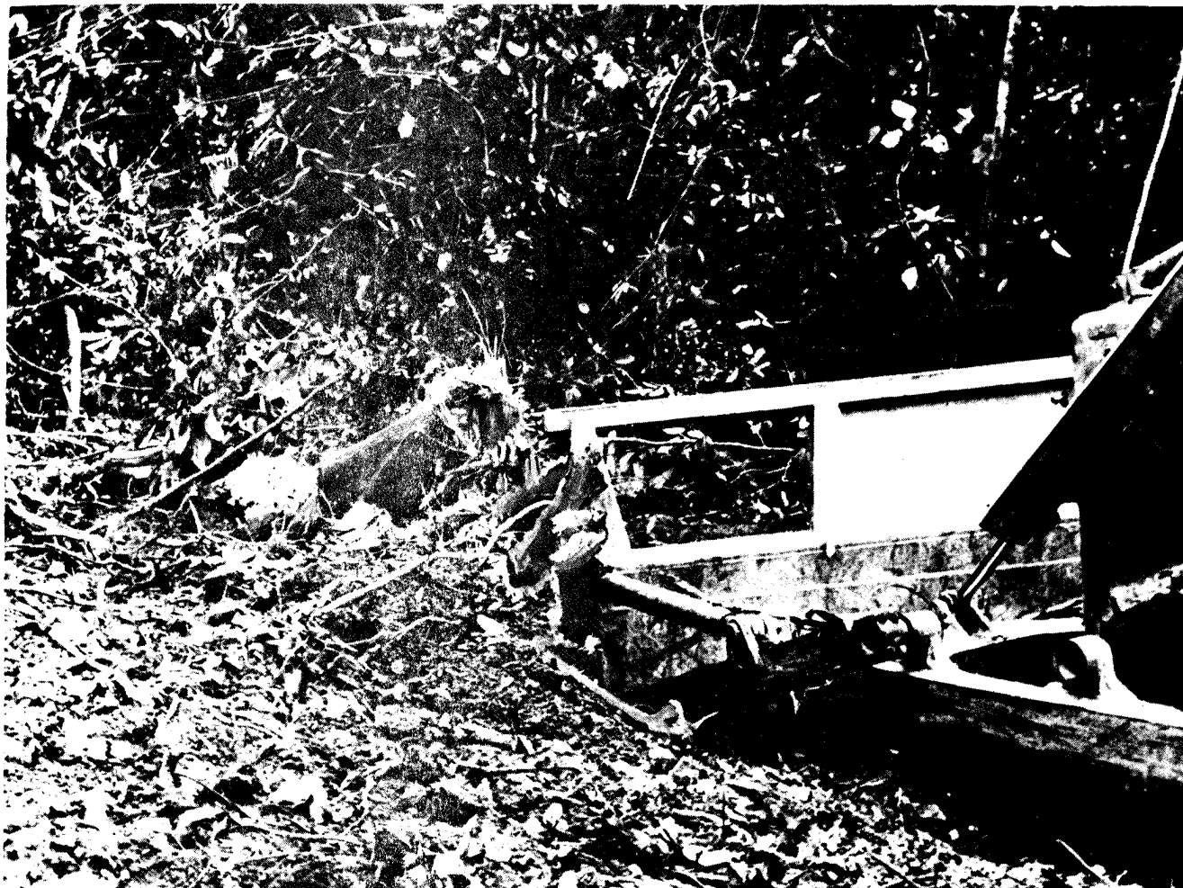
Figure 3-27. Rome K/G blade in a tilted position shearing a stump below ground level.
