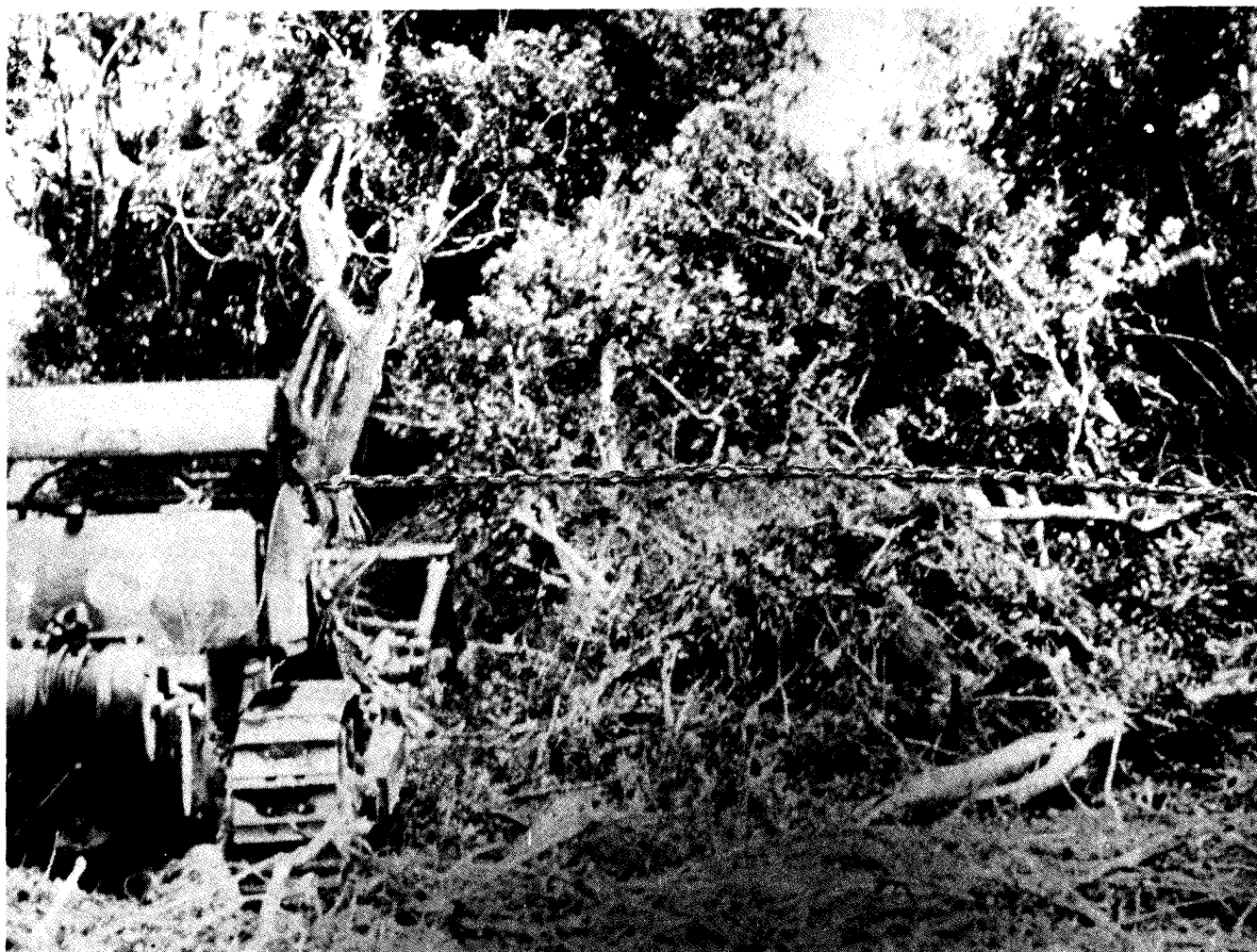
Figure 3-12. Third tractor following the chain to assist on larger vegetation.
