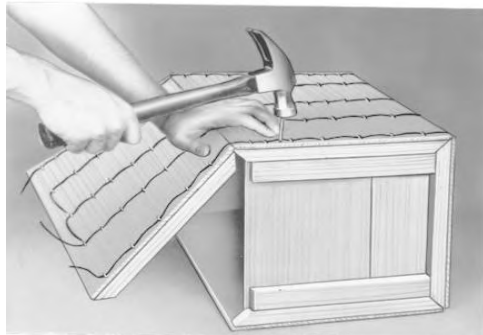
NAILING SIDE CLEATS TO ADJACENT BATTENS
