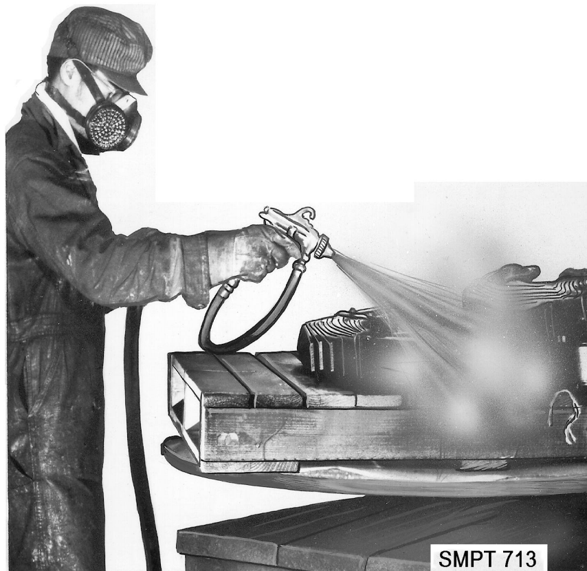
Figure 3-10. Application of preservative by spraying.
