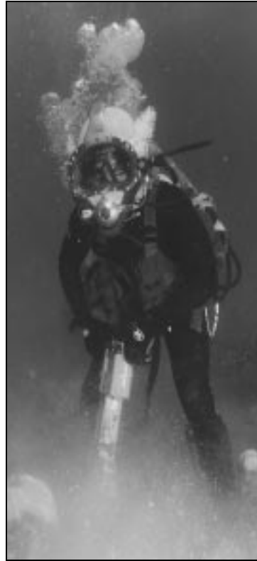
Figure 6-4. Underwater Construction Diving.
