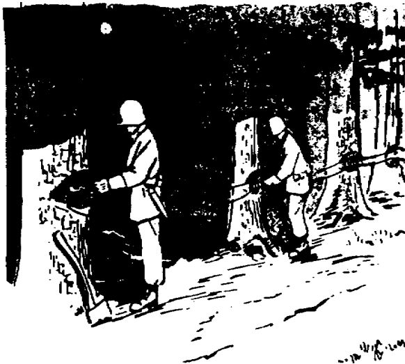
Figure 3-13. Preparing explosive charges for abatis construction.
