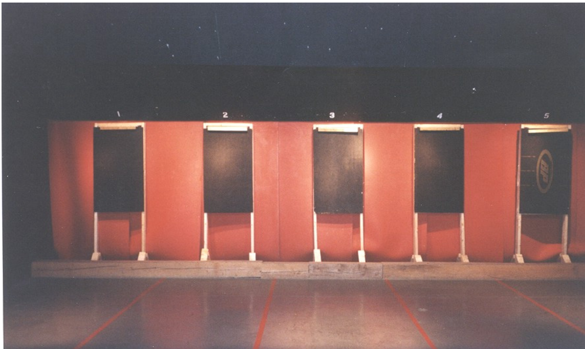
Figure 2-1: Linatex curtain with the target boards in front
