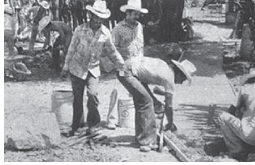
In the village of Ajoya, Mexico, over 60 families participated in building a cement walkway from the rehabilitation center to the main street.
