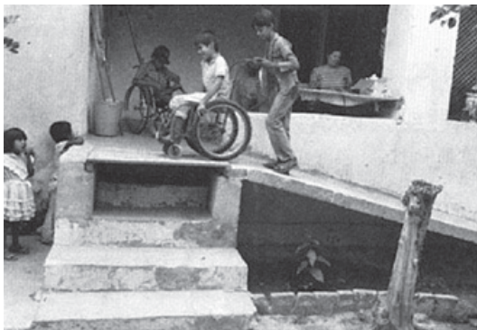
The health workers of Project Piactla built this ramp so the wheelchair riders could come into the clinic more easily. (Photo: John Fago)
