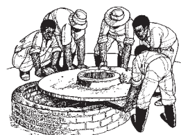
Set the well cover in place.
