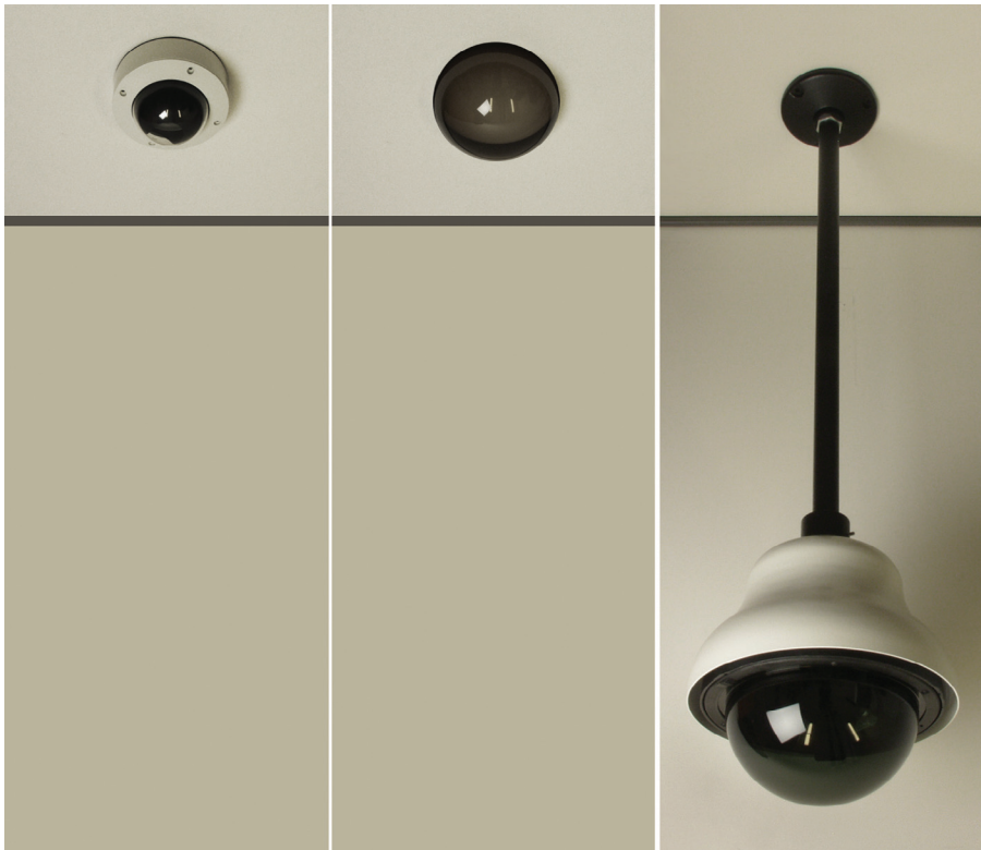
Figure 15.15 An example of a drop mount (left), a flush mount (middle), and a pendant mount (right).
