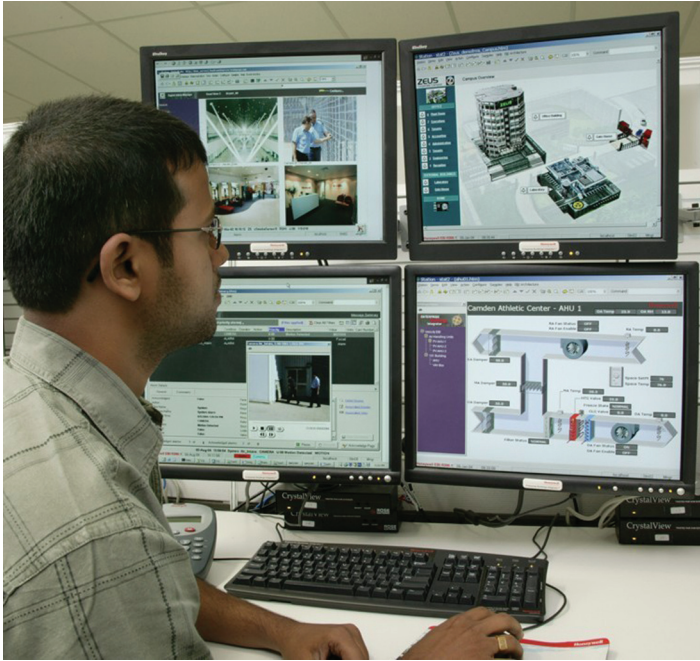
Figure 12.23 An example of a building management system that provides a single interface for monitoring a facility. The top left-hand screen provides the operator with a quad view of different camera views; the bottom left-hand screen provides an alarm summary with triggered video recordings that can be retrieved directly from an event; the top right-hand screen shows a campus graphic that enables an operator to navigate graphically throughout the system; and the bottom right-hand screen shows an air handling unit and the status and values of different controls. (Picture courtesy of Honeywell Building Solutions.)
