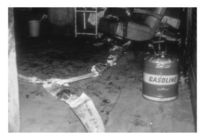
FIGURE T.8B Arson using paper as a trailer and gasoline as the accelerant.
