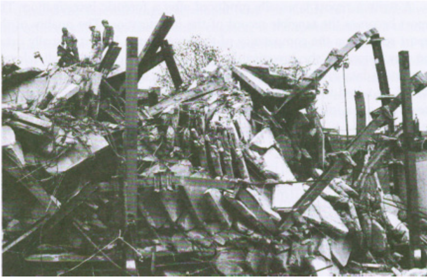
Figure 1.4 L'Ambiance Plaza, Bridgeport, Connecticut. This project collapsed during construction in April 1987, killing 28 construction workers. Useful evidence is often destroyed during the rescue efforts after such an accident [USDC/NBS 1987, Scribner and Culver 1988].
