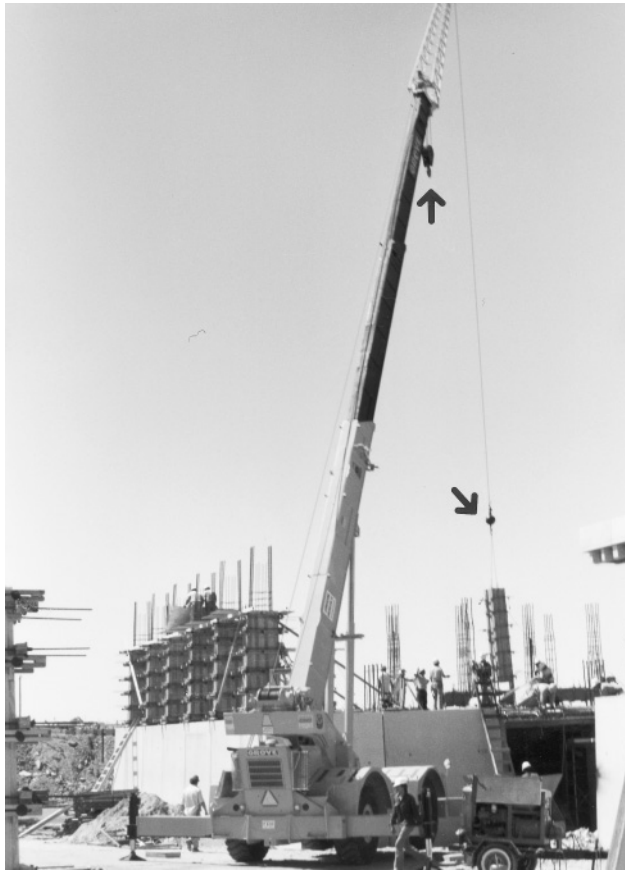
Figure 4.18 The extendible boom crane in use. Note the two cable and block systems, with the outer one being in use at this time.
