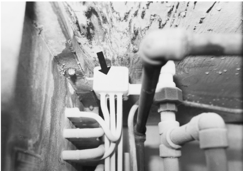
Figure 4.16 The ammonia refrigeration junction, which had been constructed from rectangular tubing, and which failed to stand up to service.
