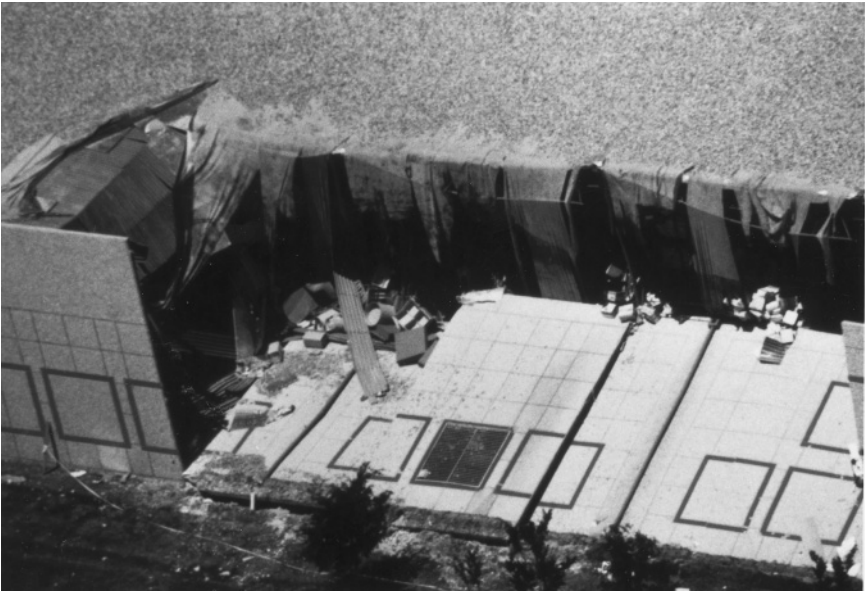
Figure 8.3 Roof and wall collapse from rain-water ponding.
