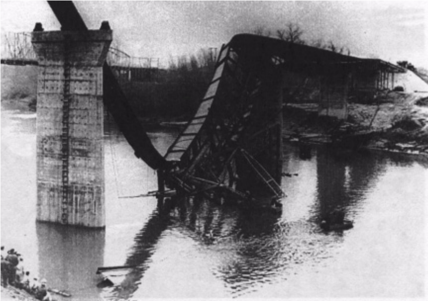
Figure 8.2 Collapse of Brazos River Bridge, Texas.
