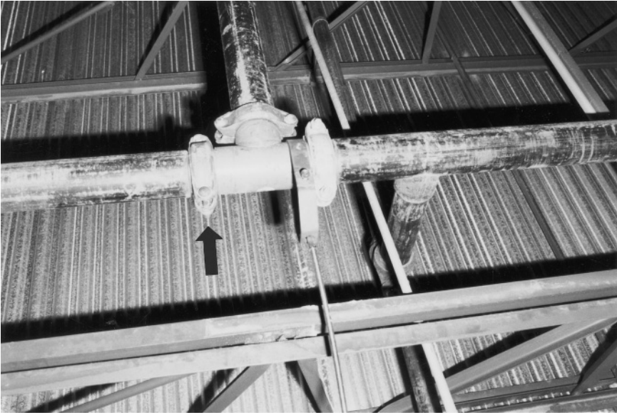
Figure 4.14 Area where a water coupling failed, allowing high pressure water to damage a building containing paper products. The arrow indicates the replacement coupling.
