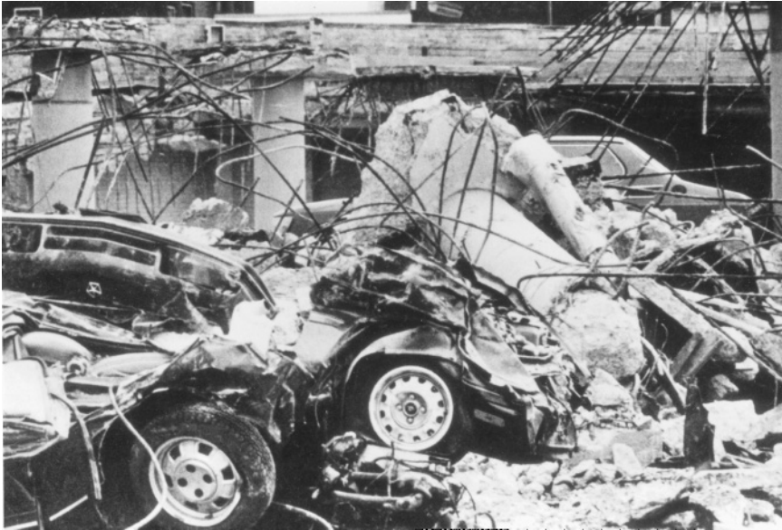
Figure 2.7 Collapse of a parking structure caused by corrosion, concealed beneath a new layer of asphaltic paving. (Courtesy of Rath, Rath & Johnson, Inc.)
