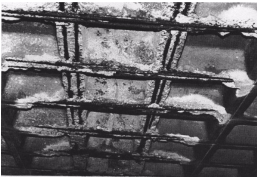
Figure 8.4 Severe deterioration at underside of parking garage slab.
