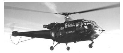
Type Accommodation Armament Maximum Speed Maximum Range Maximum Take-off Weight Length Turbine-driven general purpose helicopter Pilot plus 6 Assorted guns, missiles, or rockets 113 knots/h 340 knots 2,200 kg 12.84 m
