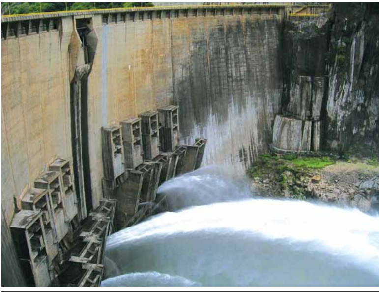
Cahora Bassa Dam
