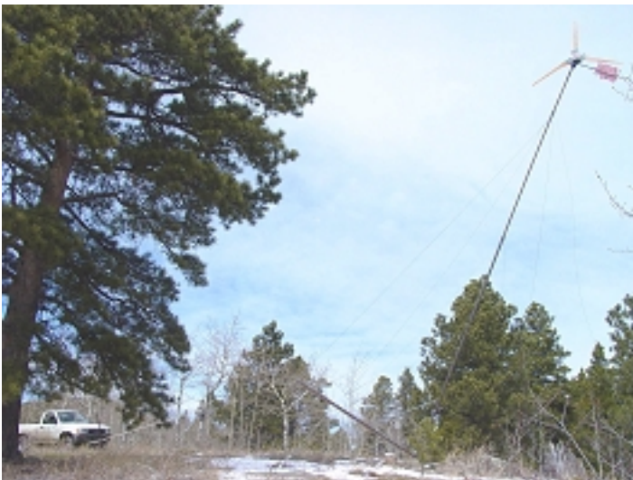
A 40-foot tilt-up tower being raised via pickup truck and gin pole. Colorado, USA
