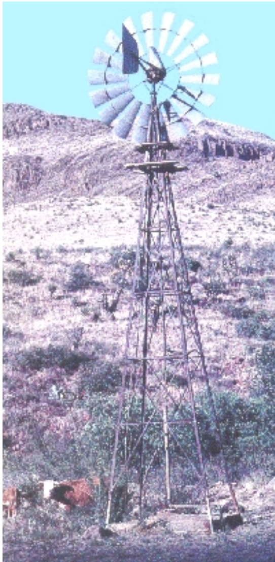
A typical Aermotor water pumping windmill, still common and in operation all over the American West. Photo courtesy of DeanBennett.com, Denver, CO. This company sells all the replacement parts to keep these beautiful old machines running, and also sells new waterpumping windmills.
