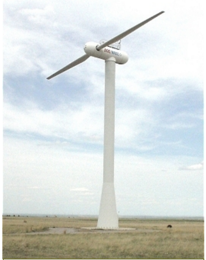
600 kW utility-scale Advanced Research Turbine at NREL’s National Wind Technology Center near Golden, CO, USA. Note how the variable-pitch blades are positioned so they can’t make power—the turbine is shut down and can’t spin. Photo by the author.
