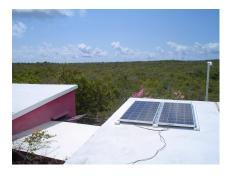
The first step is to mount the photovoltaic panels (ex. Kyocera KC130). These can be bolted to a roof or wall, or mounted on a frame in the yard. The ideal mount will point the panels at true south, not magnetic south, and titled at an angle similar to your latitude. In winter, you will get more gain if you tilt latitude +15 degree (ex. 44+15=59 degrees), in summer, latitude -15 degrees (ex. 44-15=29 degrees). Spring and fall will use straight latitude as the angle (ex. 44 degrees).
