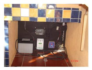
The wiring from the PV panels into the house, where the charge controller (Xantrex C-35, white box in picture above) is located, needs to be of a sufficient size to handle the current with minimal voltage loss. A 12v 130 watt panel, 100' from the charge controller, should have a 3 awg wire connecting it. At 100v (five panels in series), a 12awg wire would be sufficient. The goal is a 3% or less voltage drop. See the wire size calculator at http://www.powerstream.com/Wire\_Size.htm
