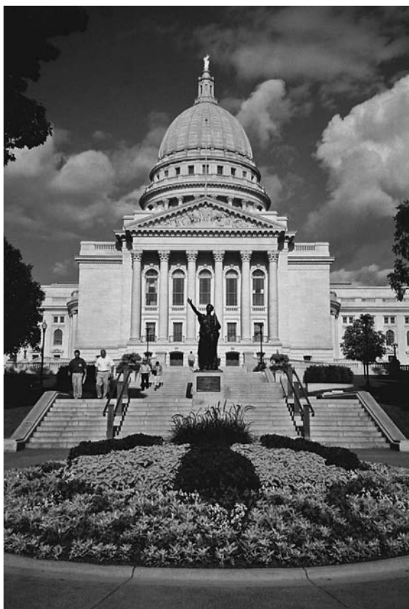
Figure 10-6 ■ Government buildings are key assets that require protection.
