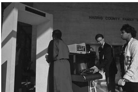
Figure 10-7 ■ Courthouse screening. Walk-through metal detector, left; X-ray scanner, right. Courtesy: Wackenhut Corp.
