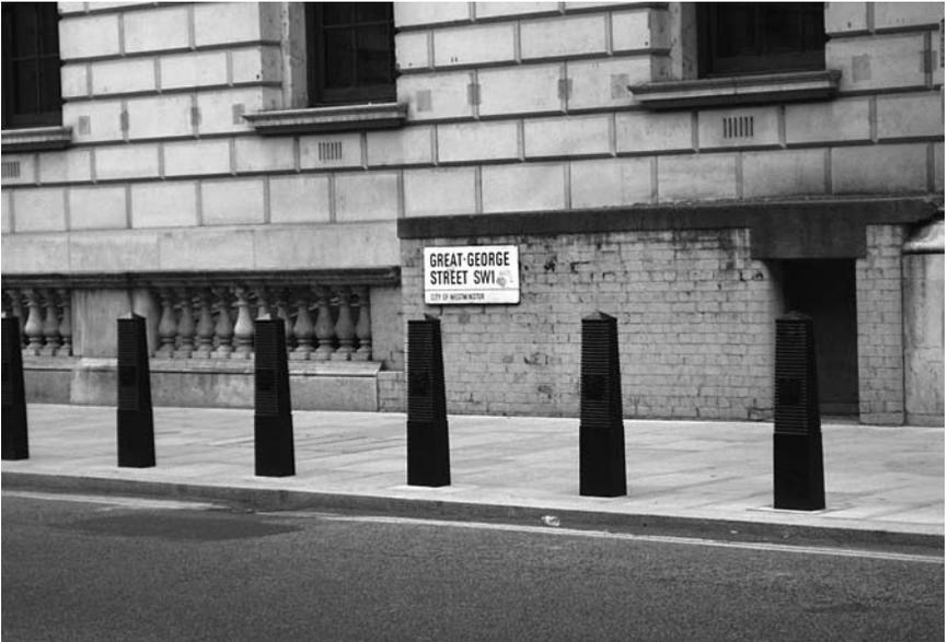
**Figure 10.7** Crash-rated bollard installed in 2008 in the Government Security Zone
