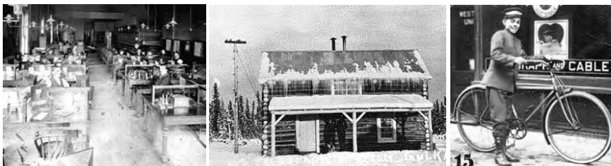
Left: The Western Union Telegraph Company grew and spread across the continent. This 1895 photograph shows the Western Union Telegraph office in Minneapolis in 1895. Middle: The Gulkana Signal Corps telegraph station in Alaska, 1910-1915. Right: A Western Union telegraph messenger, 1920. [Minnesota Historical Society photos; middle photo from the Alaska State Library, copyrights expired by date.]
