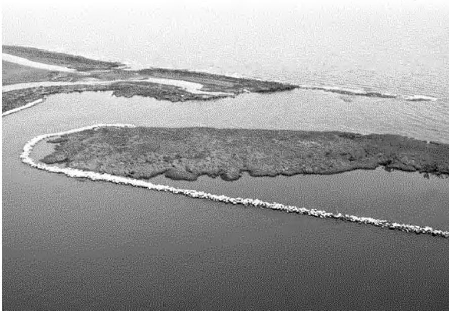
Top Left: Colonel Crear arriving for the Mississippi Delta Wildlife and Wetland Tour in the Vicksburg District in 1987. Top Right: Alligator mom in the Mississippi wetlands, just one of the many species observed during the Wetland Tour. Bottom: Erosion protection measures are illustrated where the mouth of the Mississippi River flows into the Gulf of Mexico, including banks and rock dikes, 1994. [U.S. Army Corps of Engineers news photos, released.]
