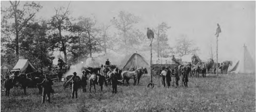
Setting up the first telegraph lines was a significant challenge. The landscape was rough and untamed, supplies were scarce, and everything had to be done by hand. Here, laborers perched atop telegraph poles like crows as the poles were being erected and the lines slung, in April 1864. Once the wires were in place, using them wasn't easy either. The typical 'telegraph station' was little more than a 25-square-foot covered wagon posted near a telegraph pole. [Library of Congress photo by Timothy O'Sullivan, copyright expired by date.]
