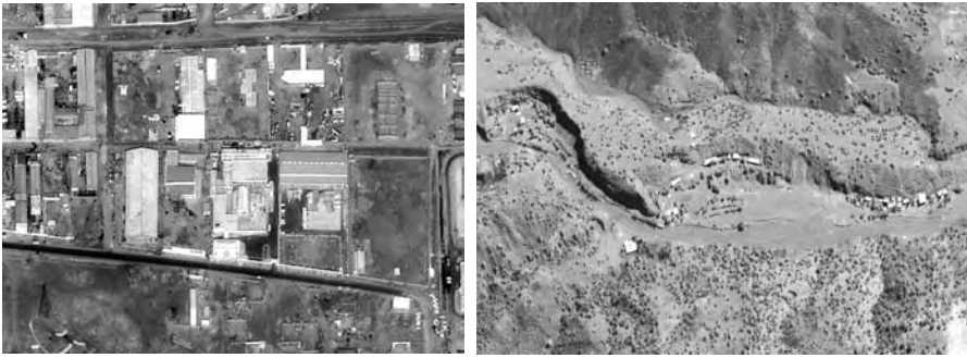
Left: U.S. surveillance photo of the Shifa Pharmaceutical Plant in the Sudan. Right: U.S. aerial photo of the Zhawar Kili Support Complex, Afghanistan. These images were used by the U.S. Secretary of Defense and General H. Shelton of the U.S. Army to brief reporters in the Pentagon on the U.S. military strike on a chemical weapons plant in the Sudan and training camps in Afghanistan. [U.S. DoD 1998 news photo, released.]
