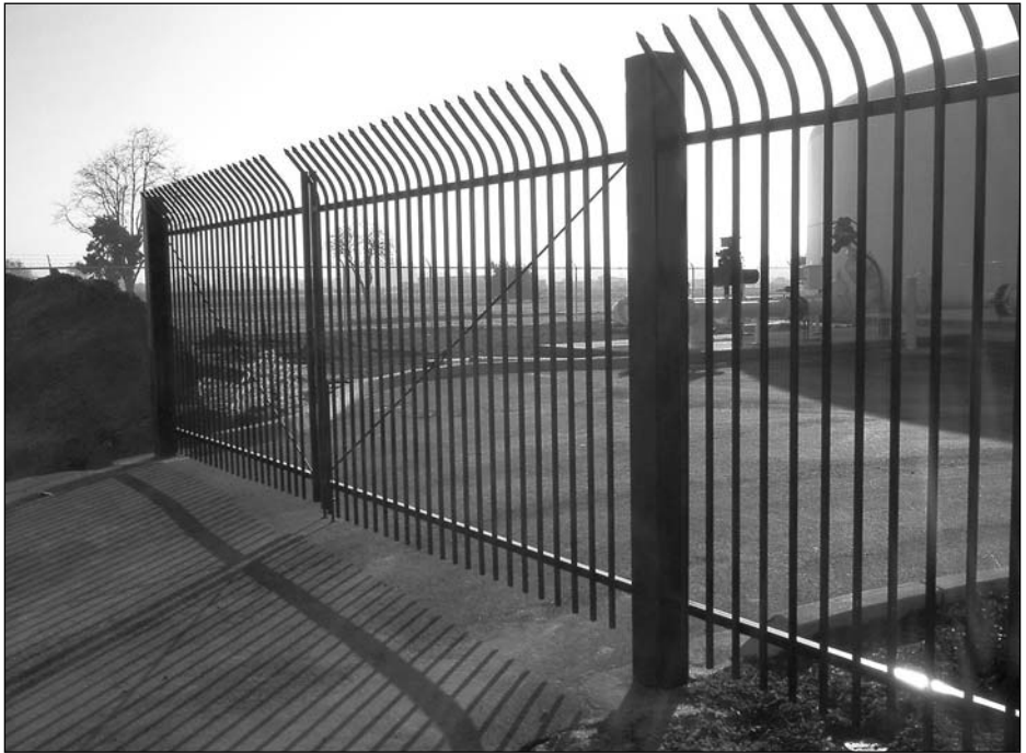
FIGURE 3-4 Wrought-iron perimeter fence
