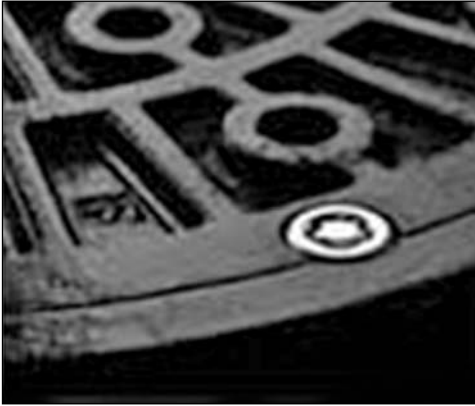
FIGURE 15.2 Manhole cover lock made by McGard, Inc. called the Intimidator™
