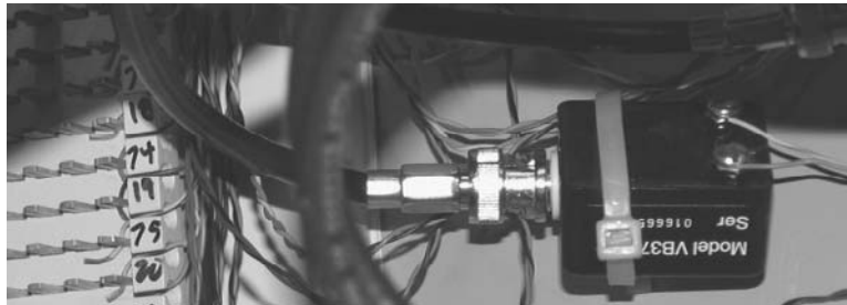
FIGURE 3-26 A Balun converting the video signal from a BNC cable into twisted pair to run the signal across the building using the existing telephone lines.
