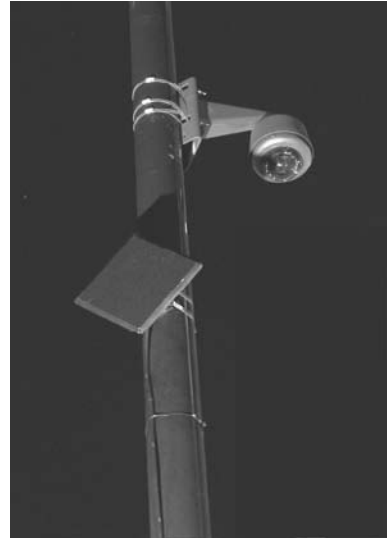
FIGURE 5-5 Directional antenna transmitting video data to a portal base station.
