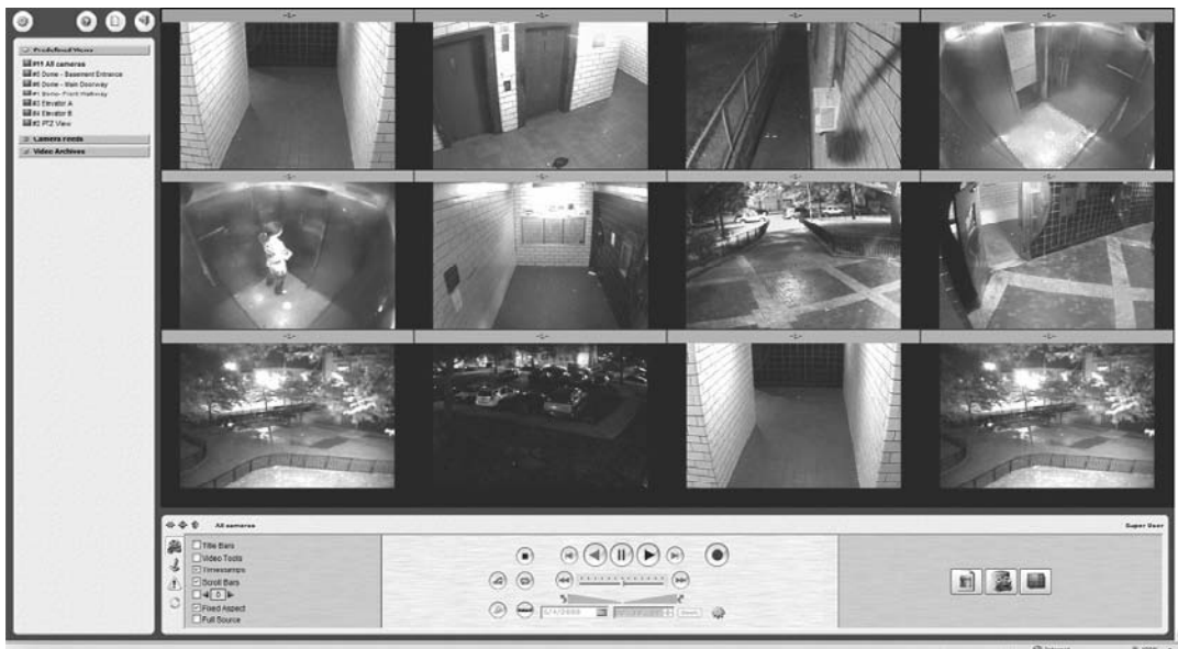
FIGURE 4-8 Using broadband over power lines speeds deployment including the mobility of elevators and areas where there is no wireless signals or data raceways.
