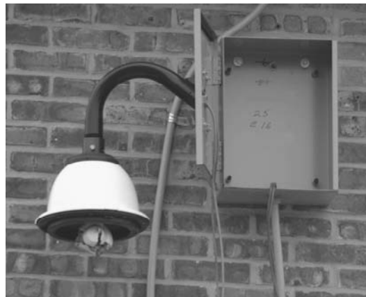
FIGURE 1-5 Not only was this camera accessible and easily destroyed, but the IP address of the network was written inside the NEMA box for all to see (not shown here).
