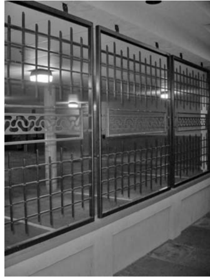
FIGURE 24.33 This garage uses high-pressure sodium vapor as its bulb choice and good ground floor protection with screening.
