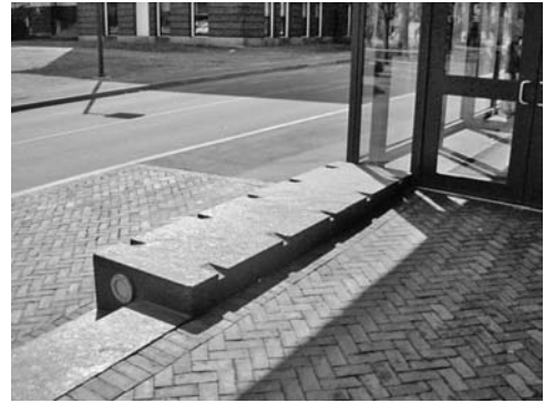
FIGURE 18.28 Incisions or notches are designed into the retaining wall prevent the surface being used by skateboarders.
