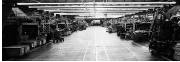
FIGURE 23.5 Sulfur lamps in a warehouse.
