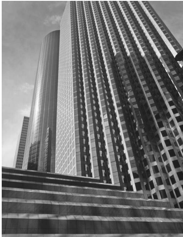
FIGURE 15.1 Building shape impacts the ability to deflect a blast wave. (Photo courtesy of iStockphoto.com.)
