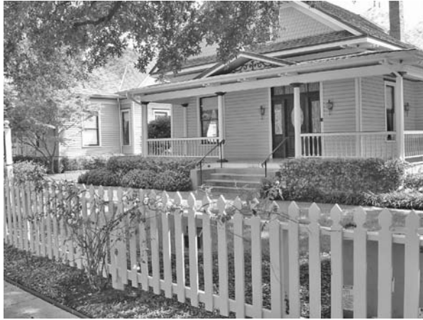
FIGURE 17.25 Picket fences and porches are the look that New Urbanists want to recreate a time and era of small towns, main streets, and a sense of community. The fencing creates a subtle form of territoriality and access control. The property looks like it is well maintained and that trespassers would be challenged.
