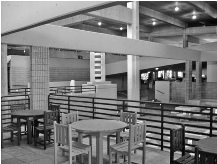
FIGURE 24.40 The placement of activities in the parking garage can create the opportunities for natural surveillance and activity support, key CPTED elements.
