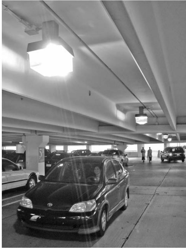
FIGURE 24.30 Lower-height ceilings should still be painted white to get as much reflection as possible. However, the structural elements will block the lighting from going sideways.
