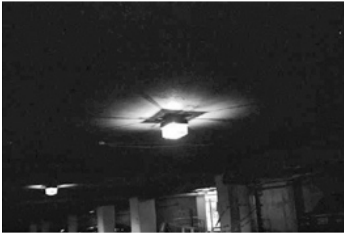
FIGURE 23.15 Ceiling before painting.
