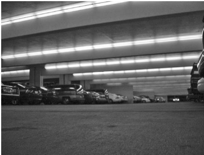
FIGURE 22.13 This parking garage used fluorescent bulbs for lighting under the structural elements.
