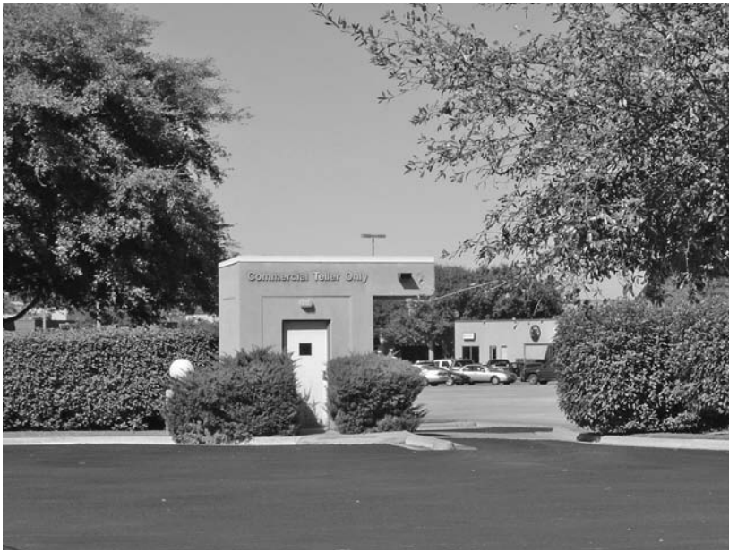
FIGURE 19.8 A remote teller window and deposit is a perfect location for a robbery. Notice the blind spots and ambush areas created by the high bushes. This would be an especially high risk at night with the cover of darkness and the element of surprise.
