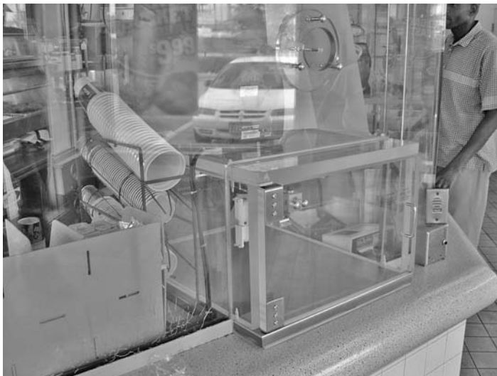
FIGURE 25.3 Bullet-resistant glazing offering protection to the employees.
