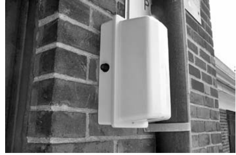
FIGURE 22.21 This porch light has a protective screen over it to reduce vandalism.
