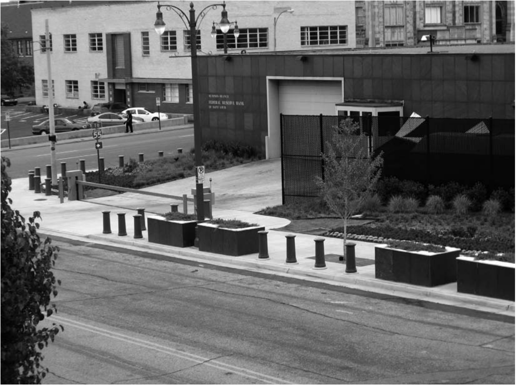
FIGURE 20.34 Street planters and bollards around the Federal Reserve Building in Memphis uses CPTED landscaping and plantings.
