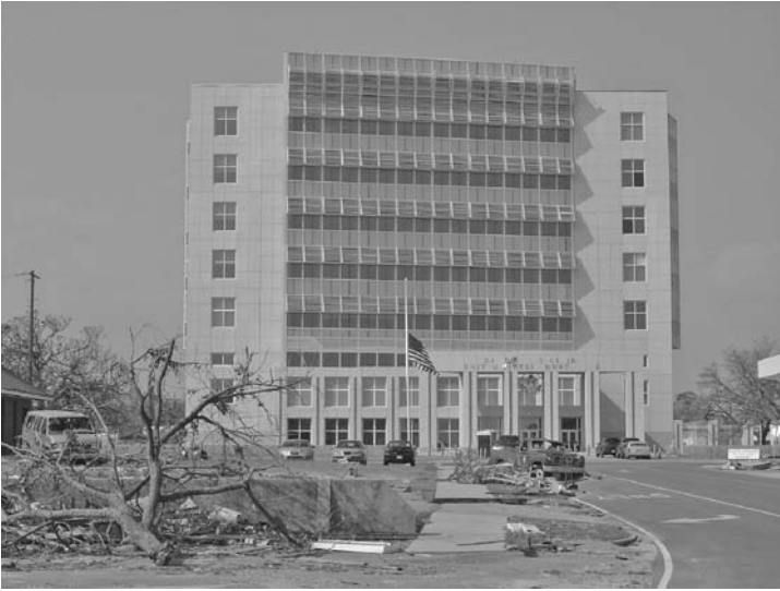
FIGURE 10.19 Gulfport, Mississippi, federal courthouse after Hurricane Katrina, undamaged by the ferocious storm because the building was designed to meet new federal security standards.
