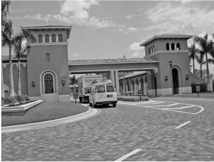
FIGURE 17.18 Many gated communities try to recreate the strong symbolic entrance of a fort or castle. It is mostly symbolic as more often than not the gates are not manned and the gate arms are not working or placed in an open position.
