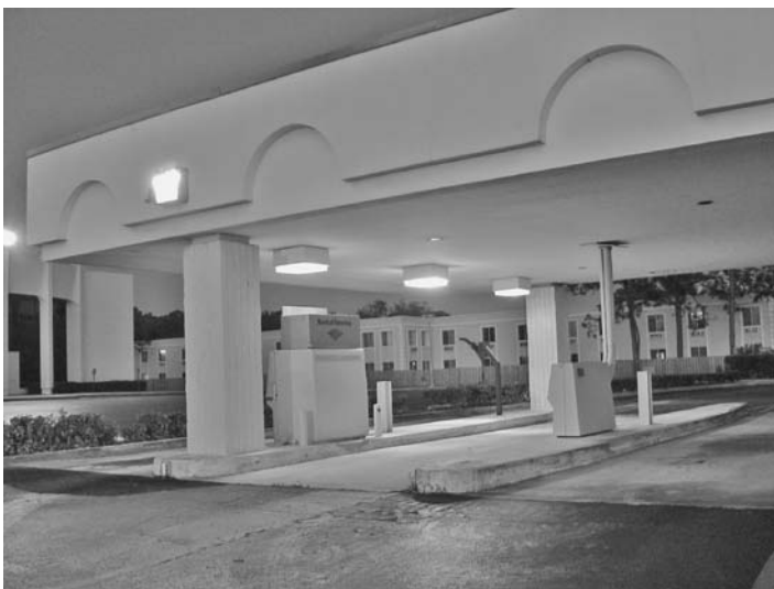
FIGURE 19.6 Lighting at a drive-thru ATM needs to be bright and consistent and avoid any hiding spaces or ambush opportunities.
