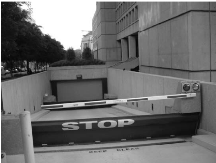
FIGURE 20.42 Mechanical barriers protect the service entrance to the FBI building in Washington DC.
