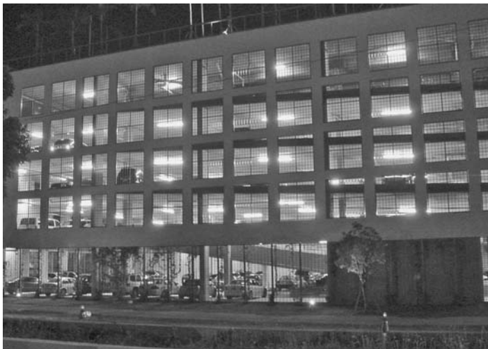
FIGURE 24.34 This garage uses fluorescent bulbs, which are typically not recommended. These bulbs are problematic in cold environments and are easily vandalized. The ground floor protection is a mesh that could easily be used as a ladder.
