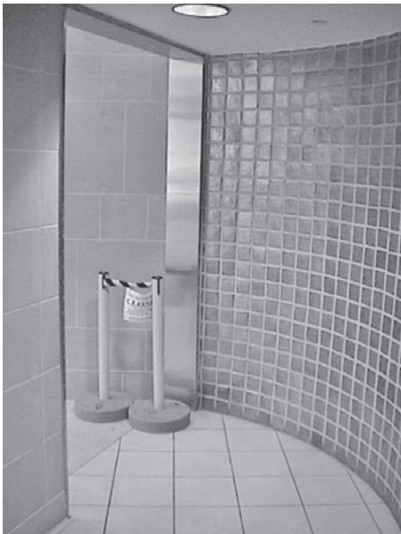
FIGURE 18.25 A lazy S design bathroom door entry.
