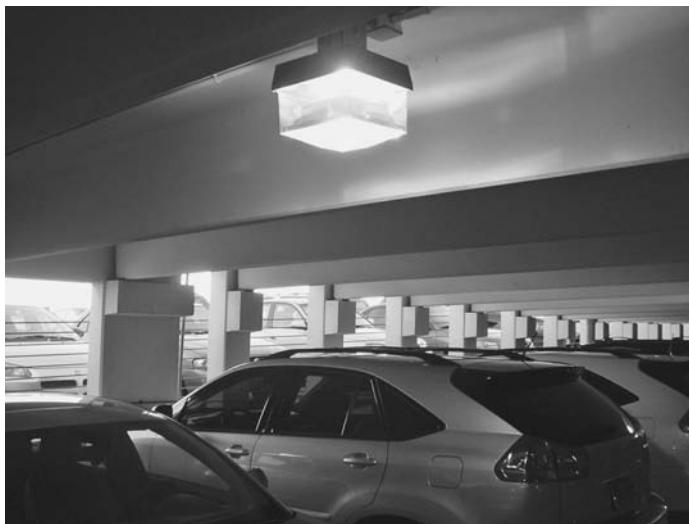
FIGURE 24.17 Open structural bays provide the best visibility. Wire cabling is used to prevent crossing through and as support against cars going through, yet allows air movement, visibility, and protection of the cars.
