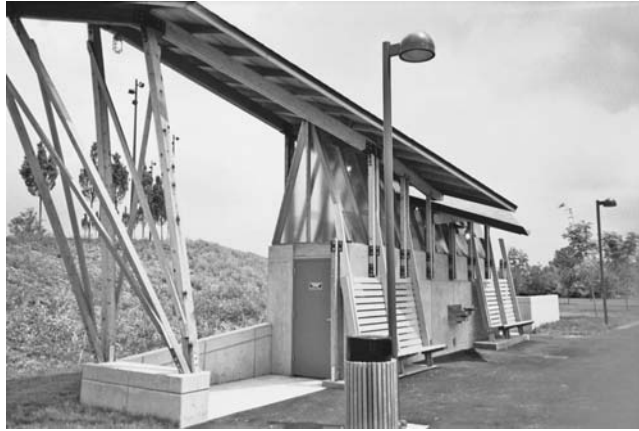
FIGURE 21.25 Park restrooms were designed to be small and very observable. The parks maintenance locked the doors after the sun went down to prevent “tearoom” activity or illicit sexual behavior.
