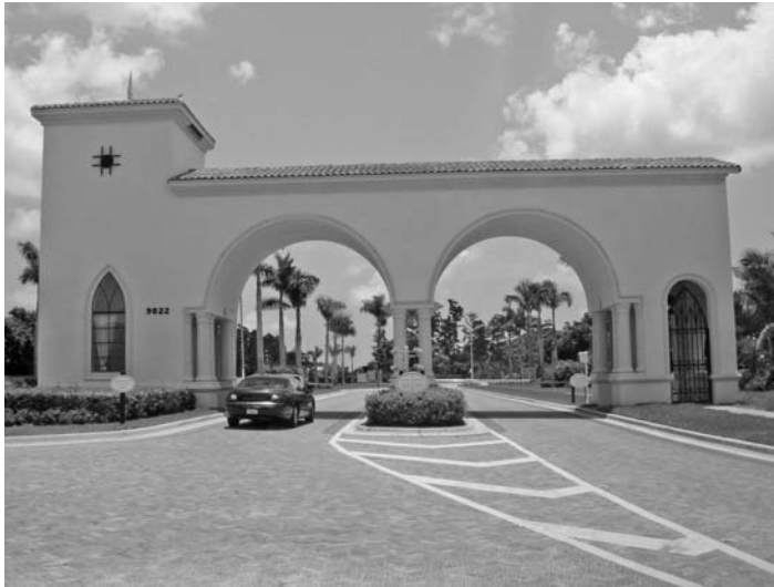
FIGURE 17.19 The gatehouse serves as a point to check visitors and vendors as to their legitimate purpose for being on-site. The residents can effortlessly pass through the right. The purpose of the gatehouse is for access control, but at what cost, and how many communities and neighborhoods can really afford this service?
