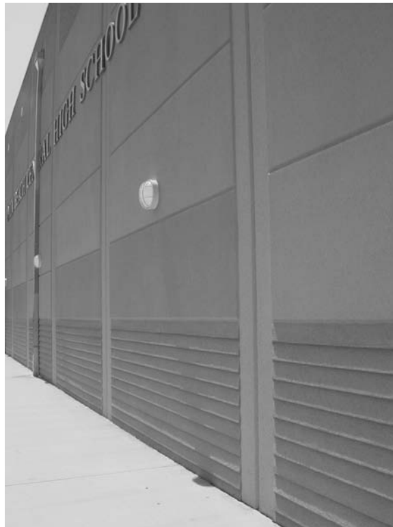
FIGURE 18.36 Textured wall painted with graffiti resistant paint removes the attractive surface to vandalize.
