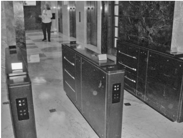
FIGURE 5.7 Optical Turnstiles used in a large office building.
