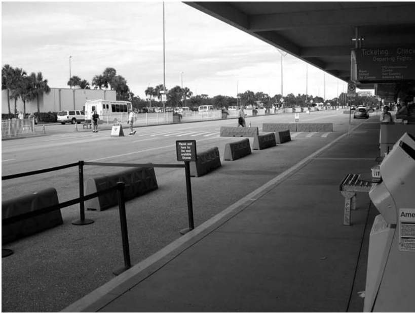
FIGURE 20.36 Ugly comes in all colors. Jersey barriers used at an airport offer no security value as they are not secured into the ground and can be easily moved by a car or pushed by several people.
