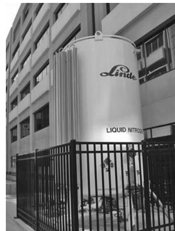
FIGURE 30.7 Liquid nitrogen container next to hospital building.
