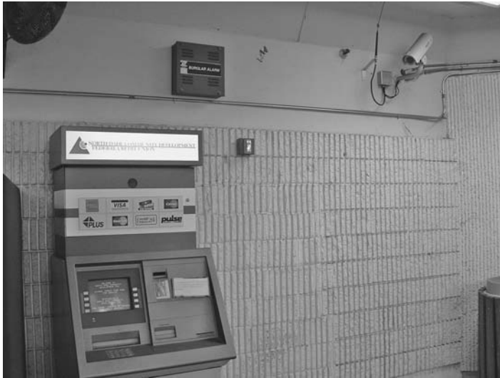
FIGURE 19.13 An ATM placed in an office lobby foyer under camera surveillance.
