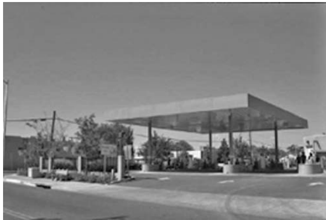
FIGURE 25.11 This gas station and store uses many CPTED design features successfully. The store is located in the corner of the site, the traffic flow is one way in and out. There is site fencing and borders to direct pedestrian traffic on the property. Bathrooms and carwash are located to the sides, in direct line of sight of the clerk.
