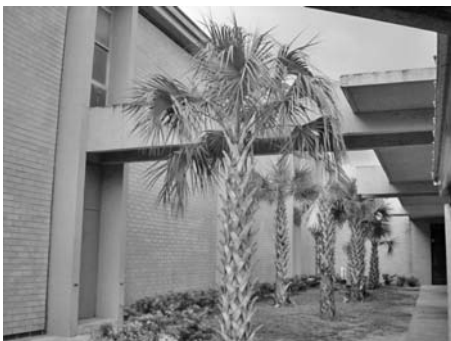
FIGURE 18.22 Catwalks access into second-floor window.
