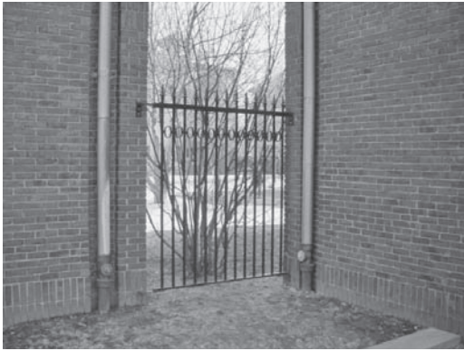
FIGURE 18.33 Fence closing the gap between two buildings and thus creating a unified security perimeter using the architectural skin and minimal fencing.
