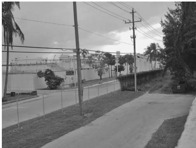
FIGURE 10.7 Perimeter fencing around the water treatment plant defines the borders.
