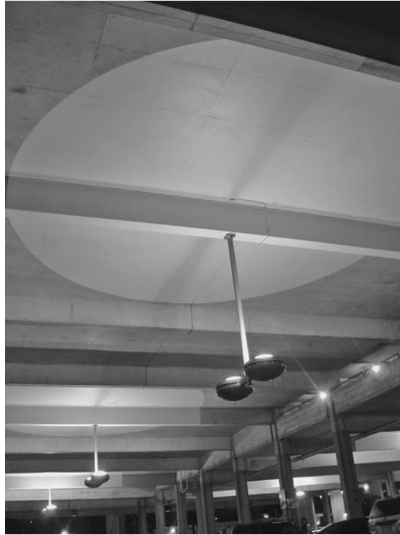
FIGURE 23.17 Example of painting ceiling to reflect light in garage.
