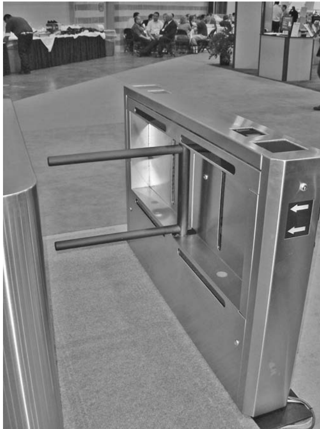
FIGURE 26.6 Example of optical turnstile.
