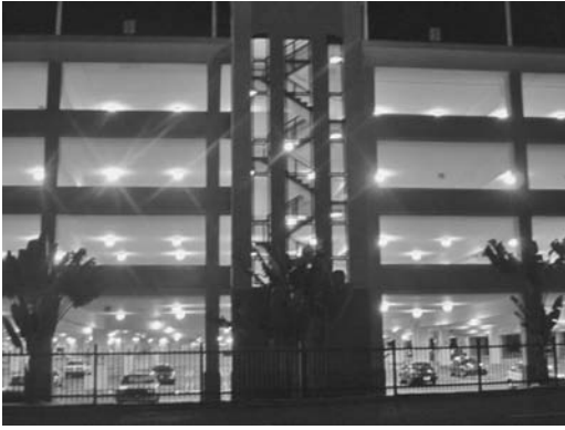
FIGURE 24.32 This garage uses all of the CPTED principles effectively, ground-level fencing for protection and access control, well-distributed metal halide fixtures, and a visible stairwell.
