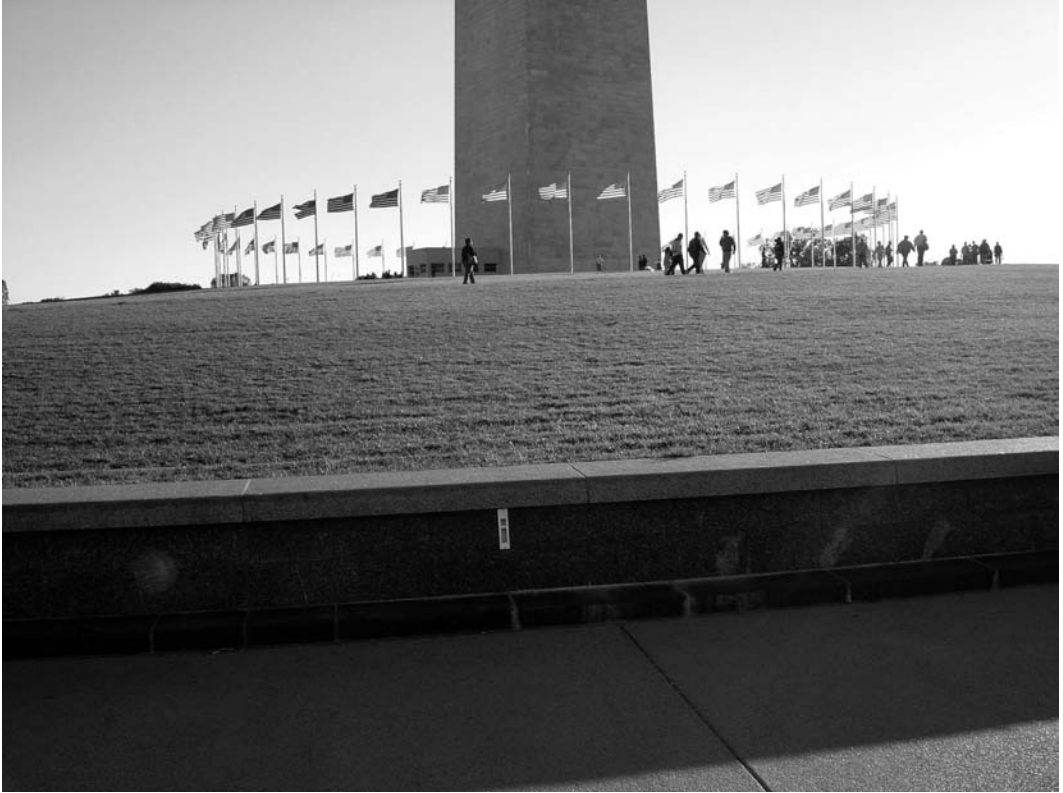
FIGURE 20.33 Washington Monument HaHa or barrier wall.
