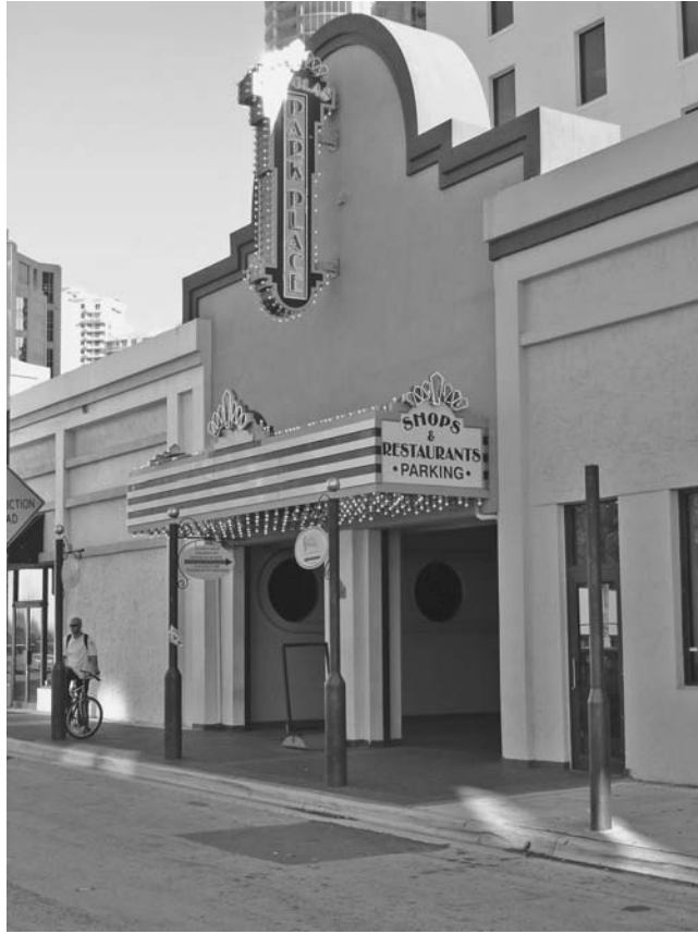
FIGURE 24.37 The garage entrance does not have to look like a garage; this one has more of a movie theater feel.
