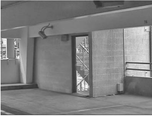
FIGURE 24.13 CCTV is watching persons that might be using the exits stairs.
