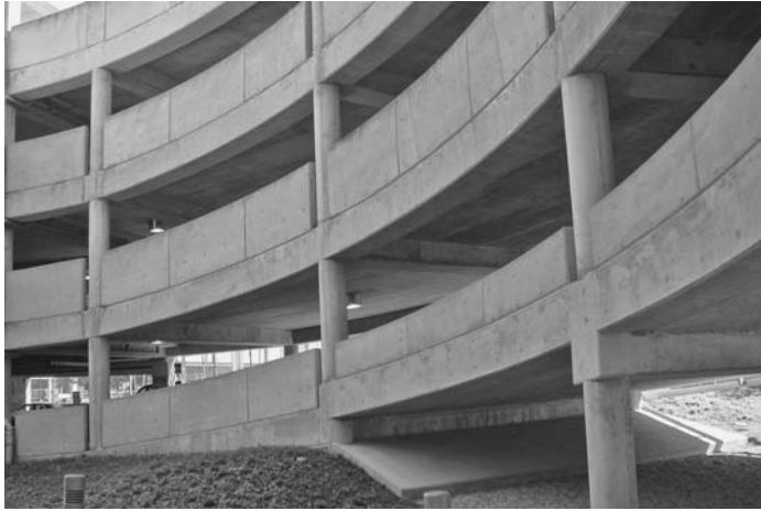
FIGURE 24.20 The use of a curved ramp system allows for the garage levels to be flat and not sloped.
