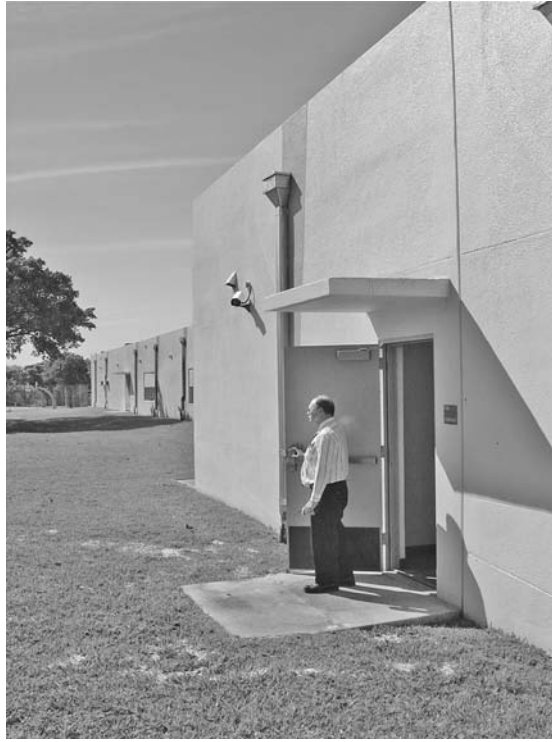
FIGURE 18.6 An exterior fire exit door to a school opens into the path of view of the CCTV camera, thus blocking the camera from seeing who is opening the door and persons entering.
