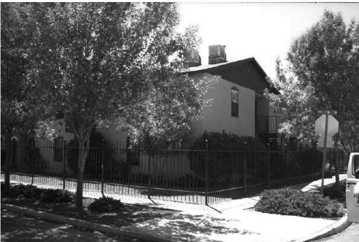
FIGURE 20.44 A perimeter fence with CPTED friendly landscaping makes for an attractive and secure border.
