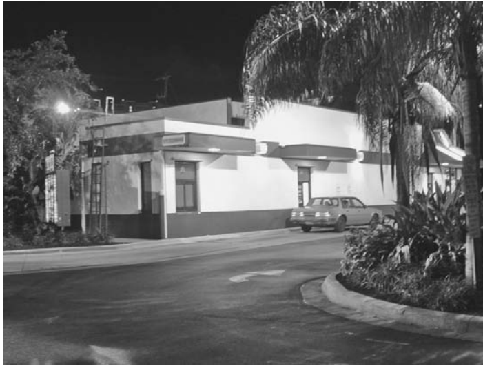
FIGURE 23.23 Good lighting quantity and quality for a restaurant with drive thru.
