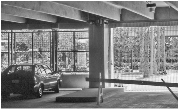
FIGURE 24.6 Secondary exits are closed with screening, and other openings are screened, creating a secure perimeter.
