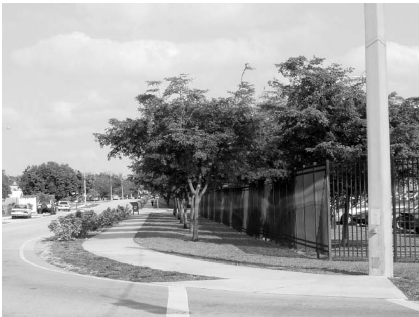
FIGURE 20.46 A perimeter fence was added around a university to create a safe boundary and control access of pedestrians and vehicles to the property.
