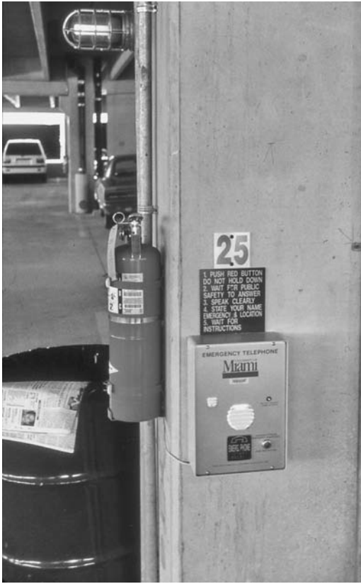
FIGURE 24.15 An example of an intercom system in a university garage and the blue light system to help direct security staff where the problem is quickly.
