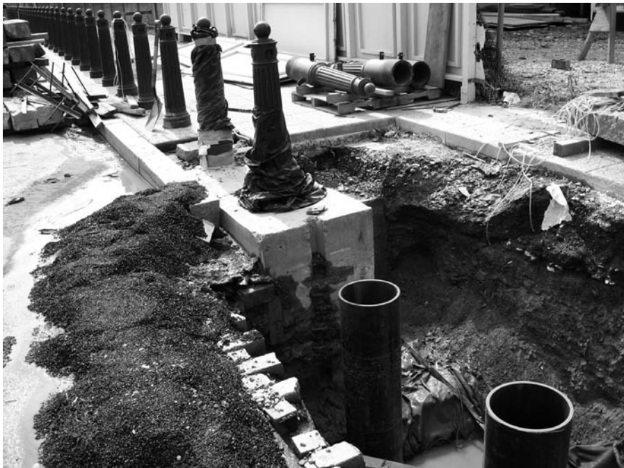
FIGURE 20.39 A good view of how the bollards are actually installed.
