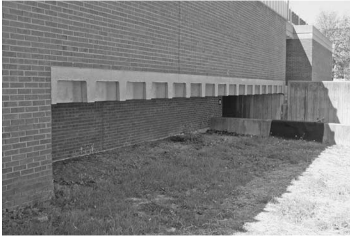
FIGURE 18.37 The alcoves in the building architecture create hiding spots and can attract persons to loiter and use as a refuge area.
