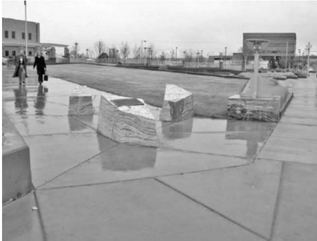
FIGURE 21.42 Art can be used as security vehicle barriers for a courthouse.
