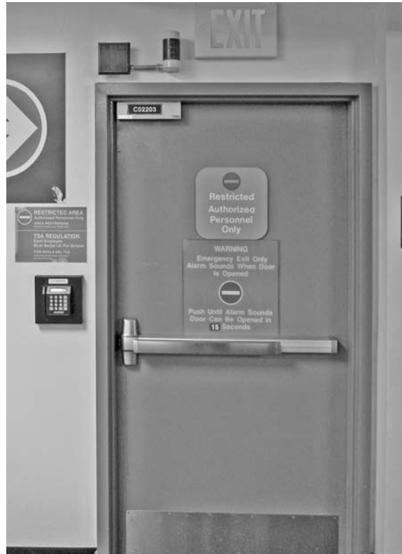
FIGURE 3.4 An example of integrated security technology and signage to make a doorway restricted.
