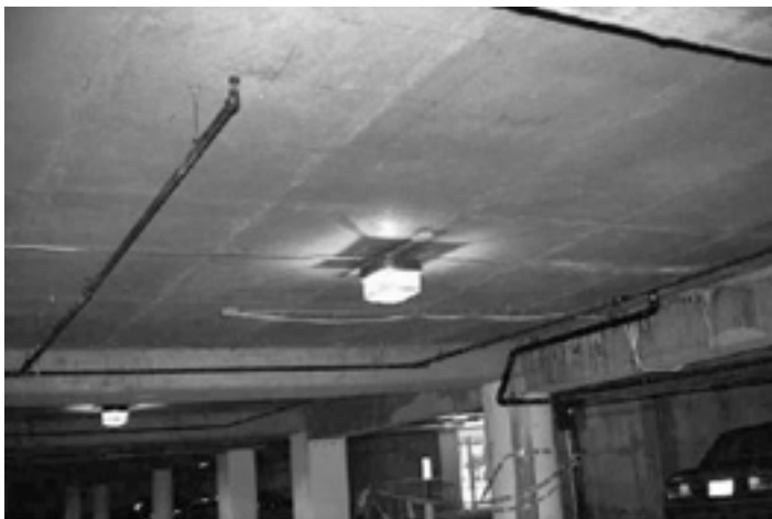
FIGURE 23.16 Ceiling after painting it white. Light reflection has greatly increased.
