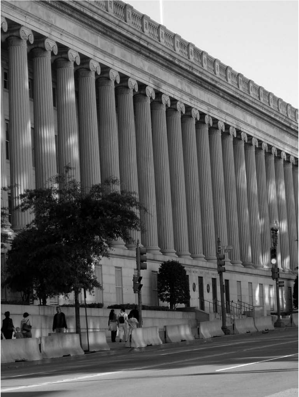
FIGURE 20.37 Jersey barriers used as an ugly and temporary solution for site protection. The barriers offer little to no site protection from a car/truck bomber.
