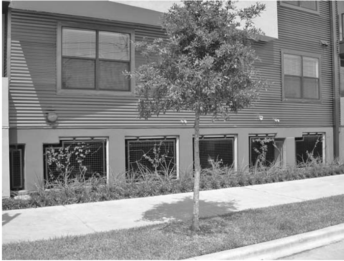
FIGURE 24.2 Subsurface parking under an apartment complex with ground level protection screens.
