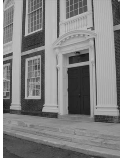
FIGURE 18.24 Noncompliant, nonaccessible entrance to a classroom building.
