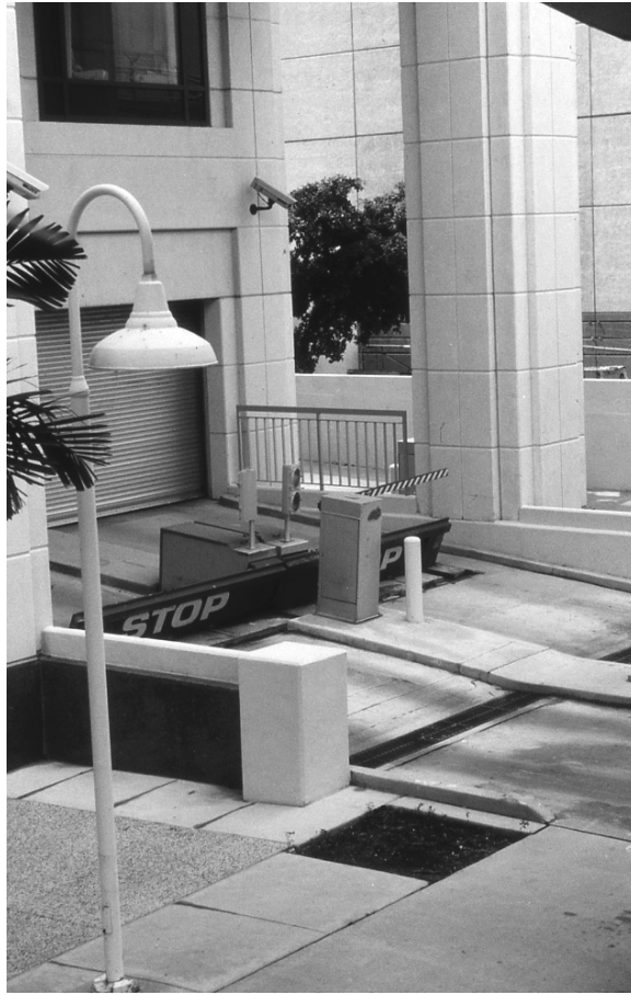
FIGURE 20.41 A combination of barriers, architectural and mechanical at the service and employee entrance of a federal office building.
