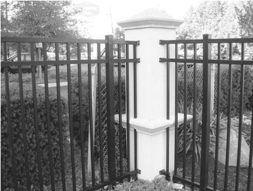
FIGURE 20.47 Good intentions for this perimeter fencing, but it has serious design flaws. The edifice on the support column only acts as a ladder, easily compromising the value of the steel picket fence.
