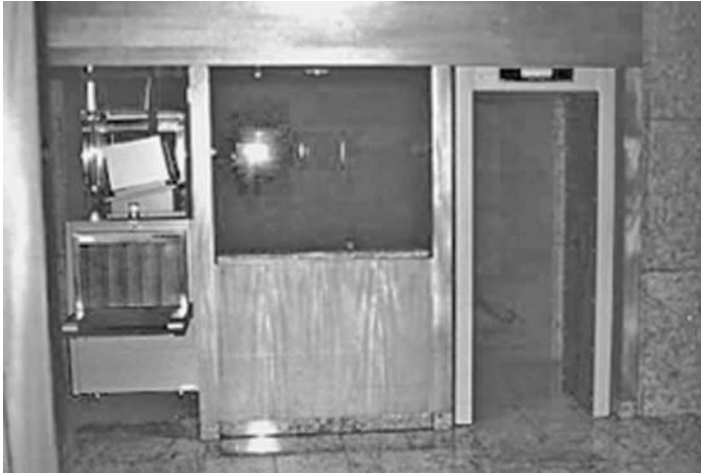
FIGURE 5.11 The lobby screening at a federal courthouse has package and person screening built into the architecture.
