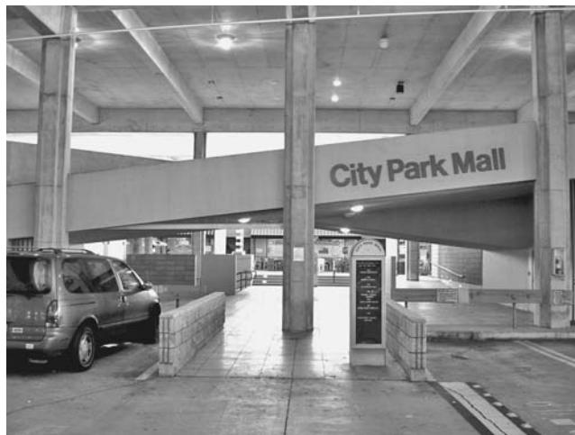
FIGURE 24.36 This garage has combined mixed uses and users, to create a facility used much of the time and by many different user groups including food court, retail, and shopping.
