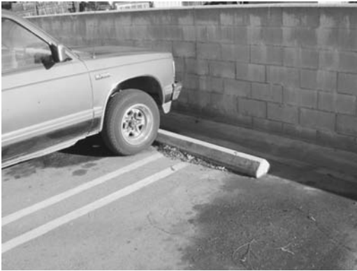
FIGURE 24.21 Wheel stops between cars may be a tripping hazard for persons not expecting an obstruction.
