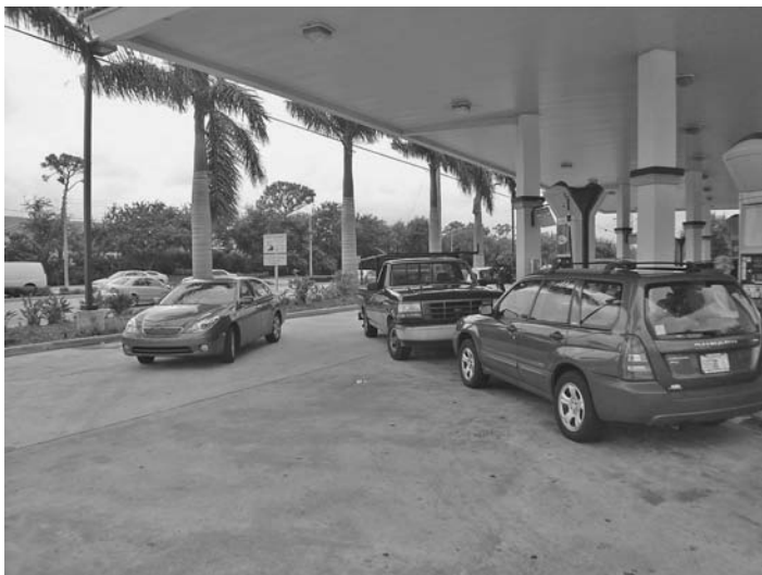
FIGURE 25.12 This gas station has conflicting travel paths for cars going to and from the pumps, and during busy times there are chaos and fights.
