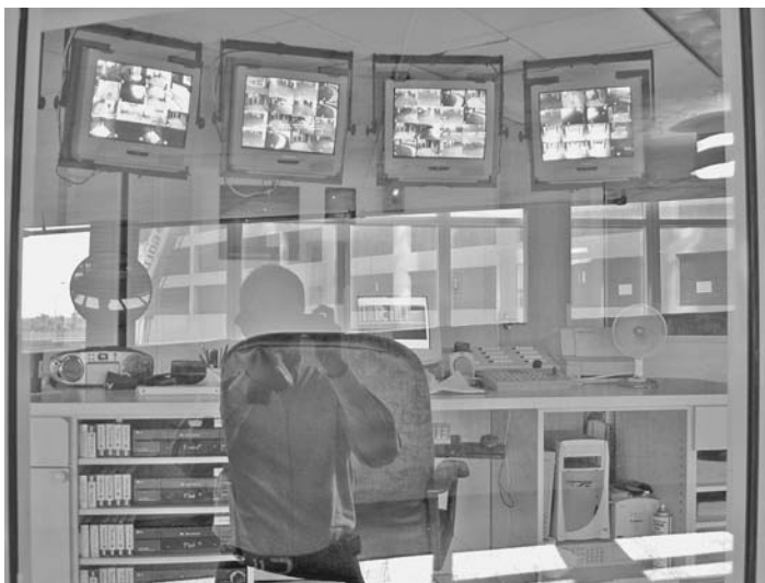
FIGURE 5.2 This control room is located in a parking garage and is remotely watching 64 cameras. Staff was nowhere to be found.
