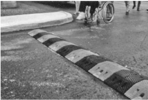
FIGURE 24.23 The speed bump is well identified, but the designer forgot to provide a curb cut in this hospital parking lot, and the patient in the wheelchair is facing a tough choice.
