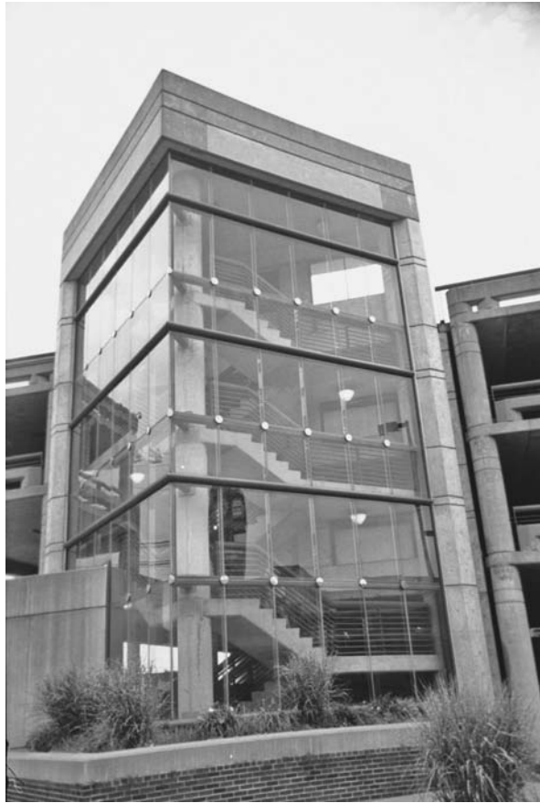
FIGURE 24.16 Exterior stairwell has good lighting and visibility.
