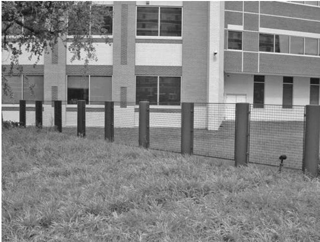
FIGURE 20.19 This office building has a monkey grass ground cover that blended nicely with the vehicle barriers. The bollards and low screening are painted green and does not draw attention to them.
