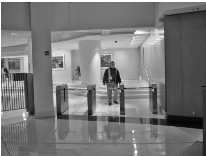
FIGURE 26.8 This office building uses optical turnstiles to allow people to exit, and there is also a mechanical gate on the far side for persons with disabilities.
