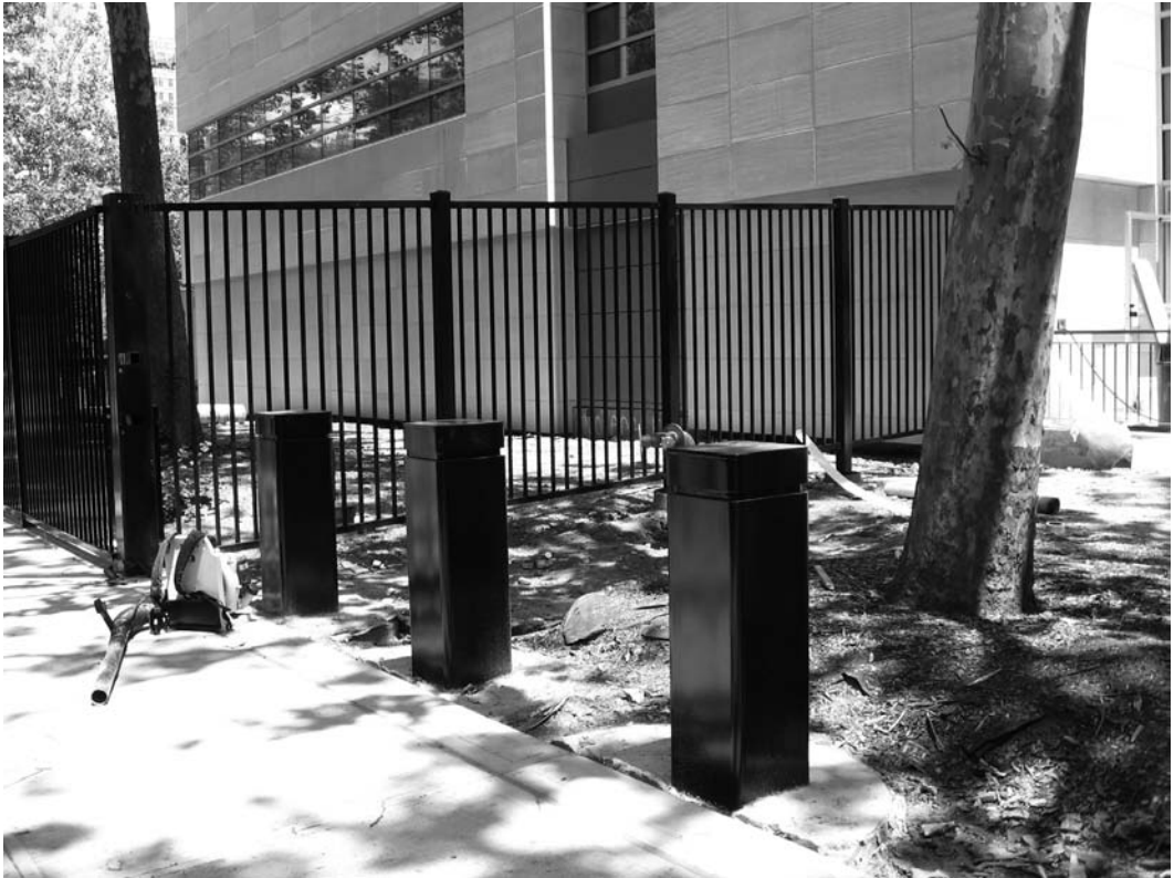
FIGURE 20.31 Crash-resistant fencing and bollards.
