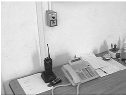
FIGURE 18.46 Communications redundancy, phones, radios, and panic alarms.
