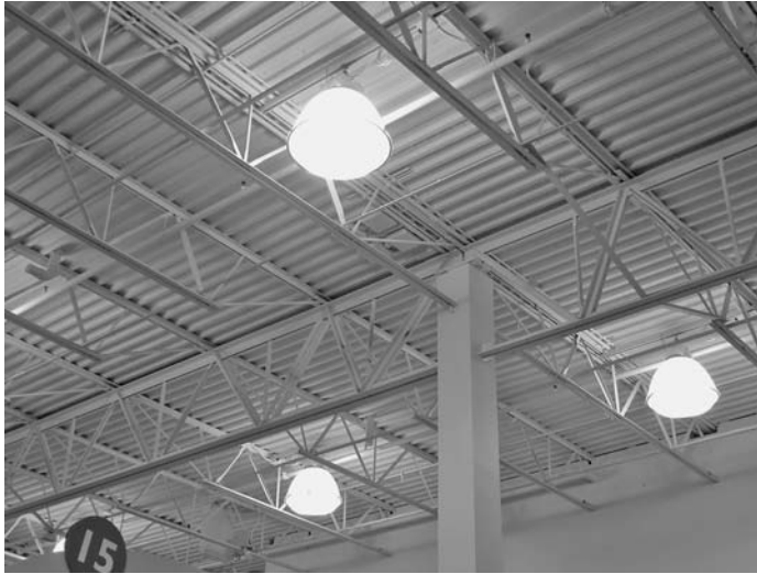
FIGURE 22.14 Mercury vapor lamps are often used in gyms and high-ceilinged department stores. Although apparently used in fewer situations across North America than before, mercury vapor is another bright industrial light source.
