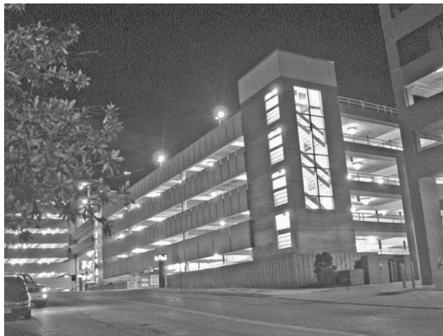
FIGURE 24.31 This garage is well lit and also has a well-designed stairwell using metal halide luminaries.
