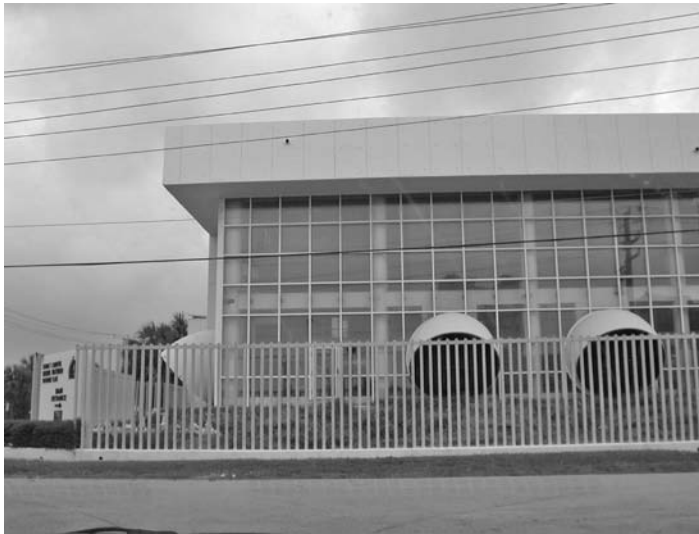
FIGURE 10.3 George T. Lohmeyer Regional Wastewater Treatment Plant perimeter fence.
