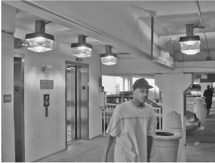
FIGURE 24.24 The lobby foyers and elevator landings should be easily identifiable from the far end of the garage; this can be facilitated by signage and lighting.
