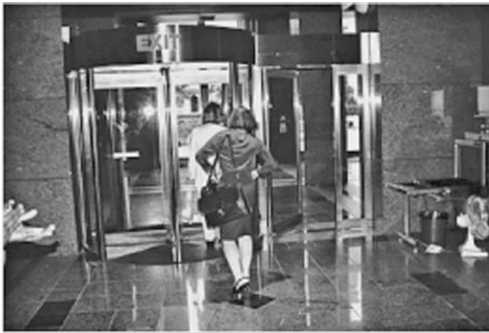
FIGURE 5.12 Revolving doors are great tools to permit controlled entrance and prevent piggybacking, but they are not friendly to wheelchairs and subsequently a glass swinging door is also provided to allow accessible entrance to persons with disabilities.
