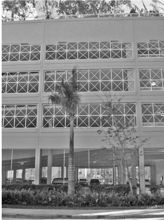
FIGURE 24.8 This garage has smart placement of trees and plantings that does not interfere with lines of sight or the ground level screening.
