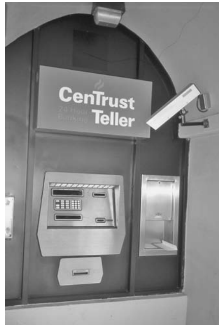
FIGURE 19.12 A well-planned ATM with lighting and CCTV coverage.
