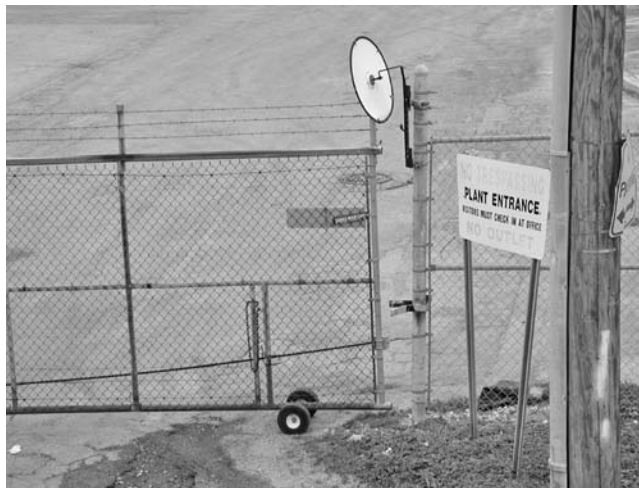
FIGURE 10.5 Plant access gate for parking and administrative office is left unlocked, undermining all of the other physical security measures.
