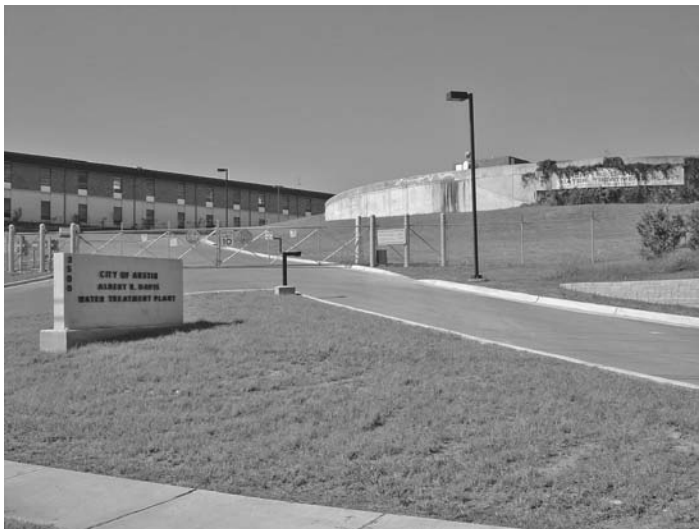
FIGURE 10.2 Water treatment plant entranceway.
