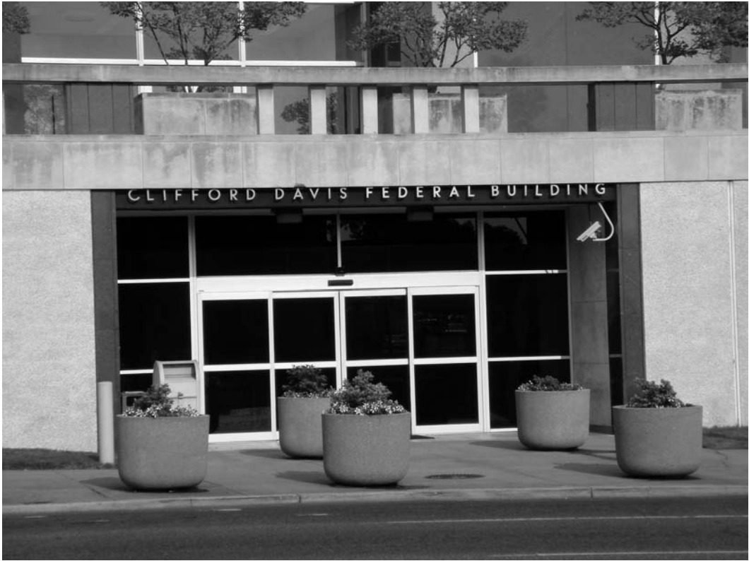
FIGURE 20.30 Planter bollards, acting as a vehicle barrier in front of a Federal Building.
