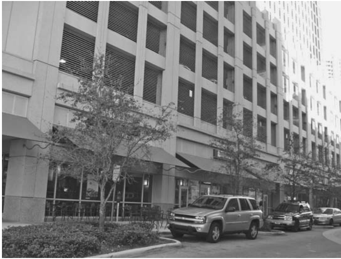
FIGURE 24.39 This garage has shops on the ground floor, but because this is an office building, the garage and most of the shops are closed on the evenings and weekends.
