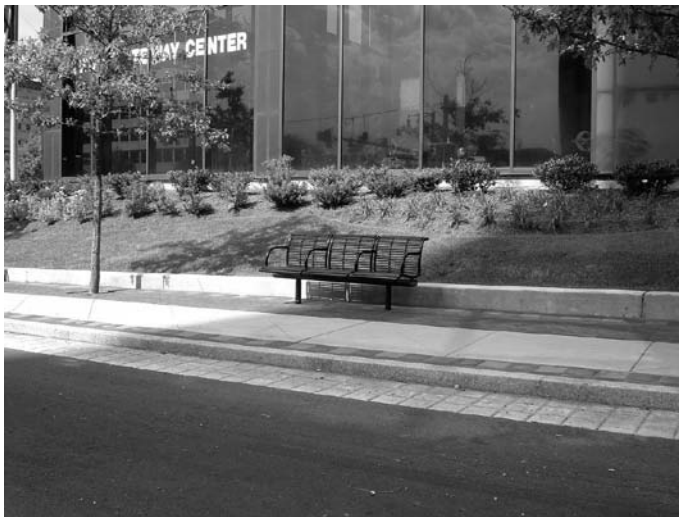
FIGURE 20.28 CPTED friendly bench with low ground cover and retaining wall that can act as a vehicle barrier.
