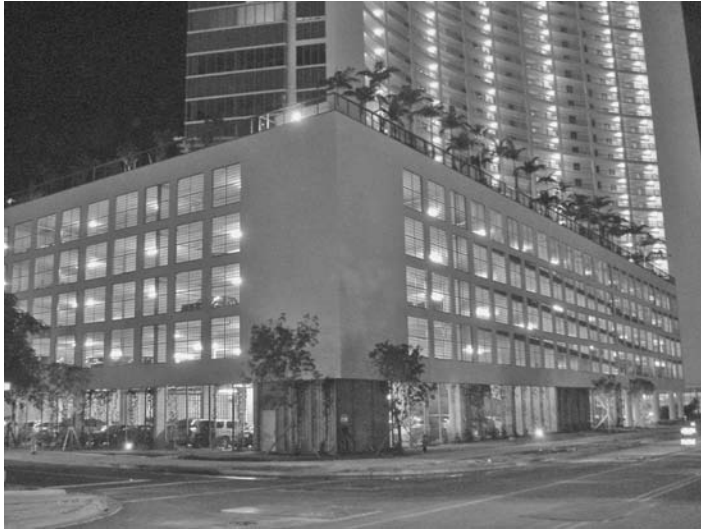
FIGURE 24.35 The garage may be lit up brightly now because this is a new building, but the openness to outside elements make the fluorescent luminaries a poor choice, considering the likelihood of severe weather and salt air in Miami.
