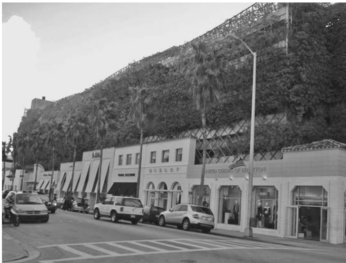
FIGURE 24.38 This garage camouflaged the garage with landscaping and plantings and celebrated its ground-floor businesses, which are open around 18 hours a day.
