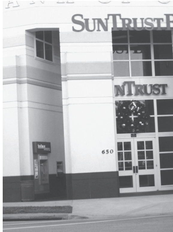
FIGURE 19.3 This ATM is shielded by structural columns at this bank, making visibility almost impossible.
