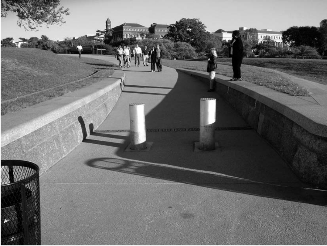
FIGURE 20.32 Vehicle barriers around the Washington Monument
