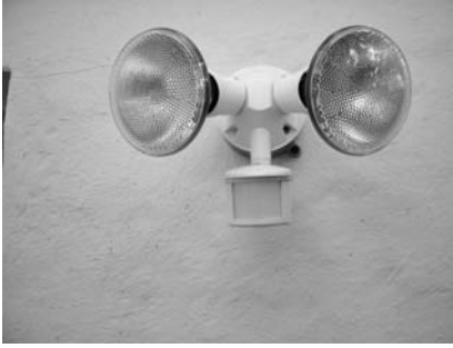
FIGURE 22.20 Flood lights are combined with a motion sensor to come on when movement is detected.
