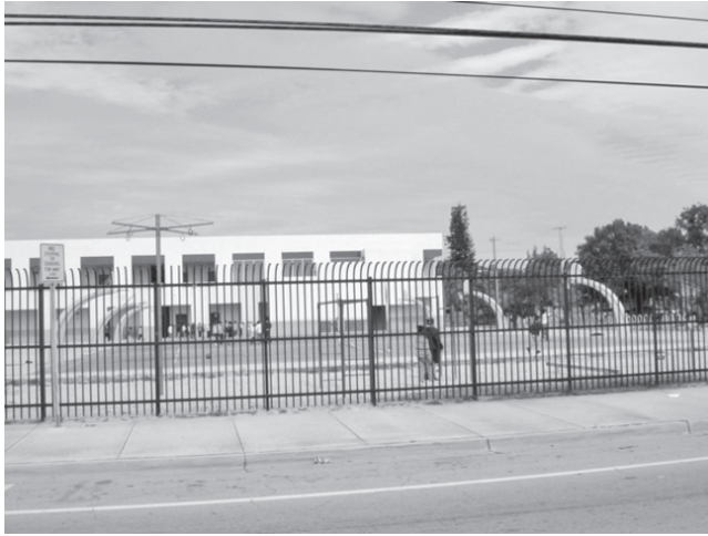
FIGURE 18.13 School boundaries are important but must not be intended to make the property look and feel like a prison. The intermediate support railing on the fence pretty much renders the security fence worthless. A juvenile could scale the fence in seconds.
