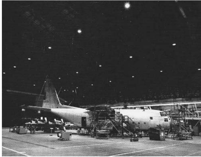
FIGURE 23.7 Hangar using sulfur lamps.
