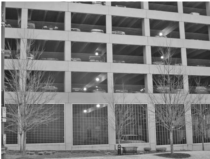
FIGURE 24.3 A Memphis parking lot with ground-level screening.
