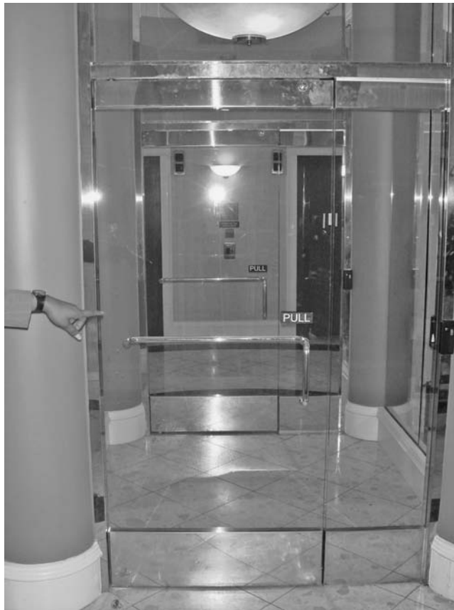
FIGURE 26.3 This office building has a security vestibule or sallyport that permits screening yet allows good surveillance and blends into the architecture.
