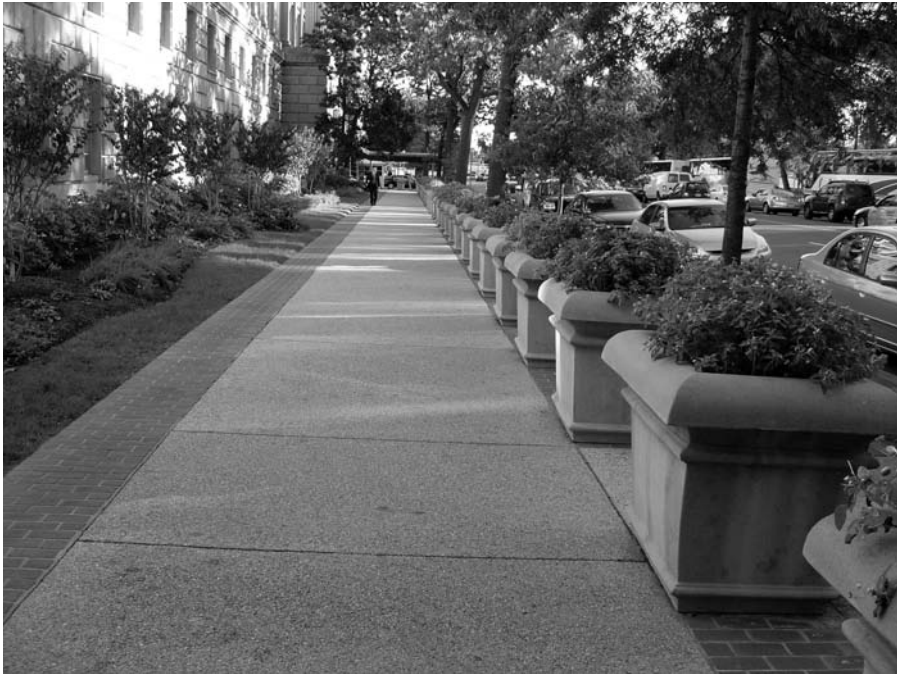
FIGURE 20.38 Security planters offer protection and a sense of territoriality around the perimeter of the property.
