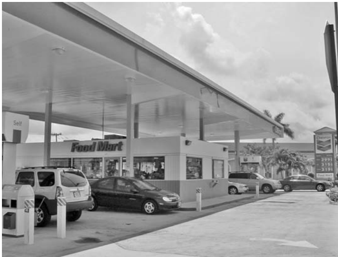
FIGURE 25.14 Windows allow visibility and surveillance of both sides and front of station and site.
