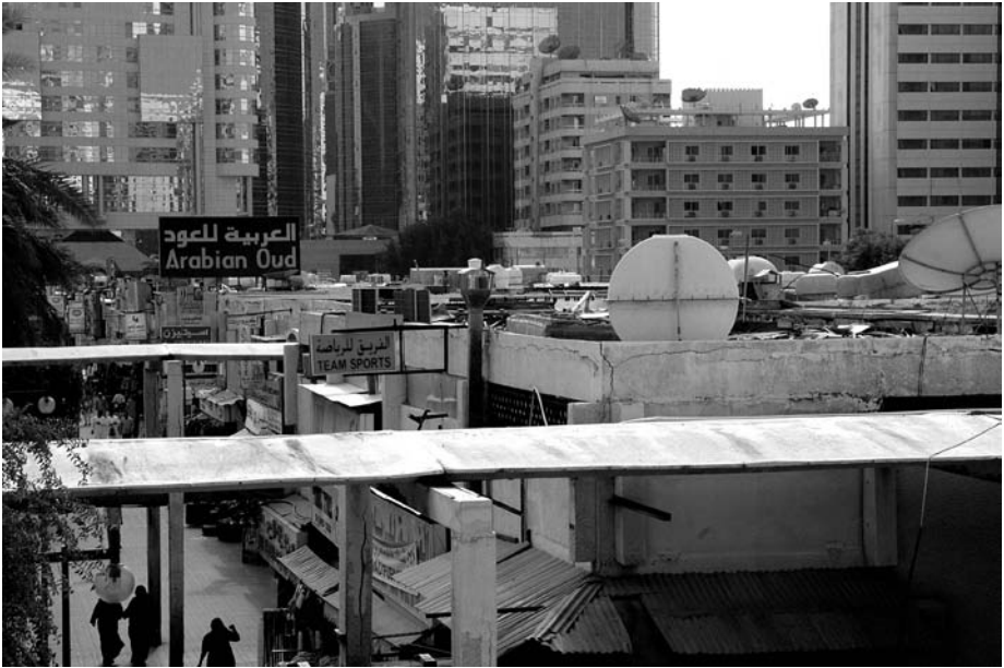
Figure 10.10. The central market prior to demolition. View from the pedestrian bridge.
