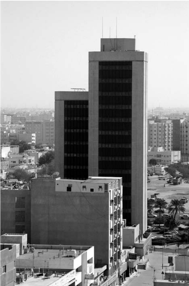
Figure 9.4. Until very recently, the Jeddah office tower was the highest structure in Doha.
