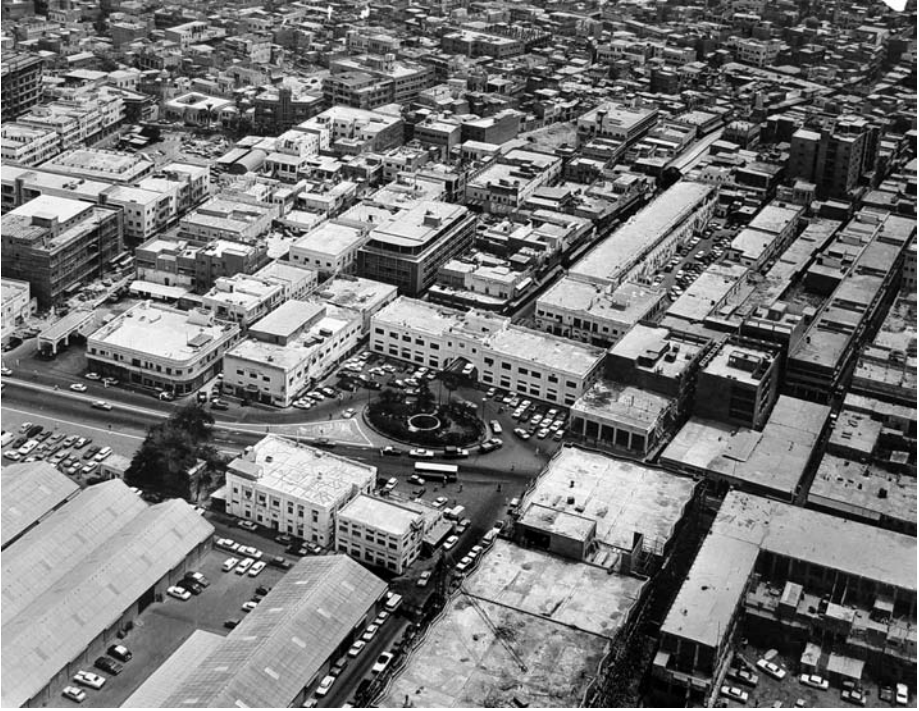
Figure 8.7a. Aerial view of Bab al-Bahrain gate showing the early political and administrative district in Manama.
