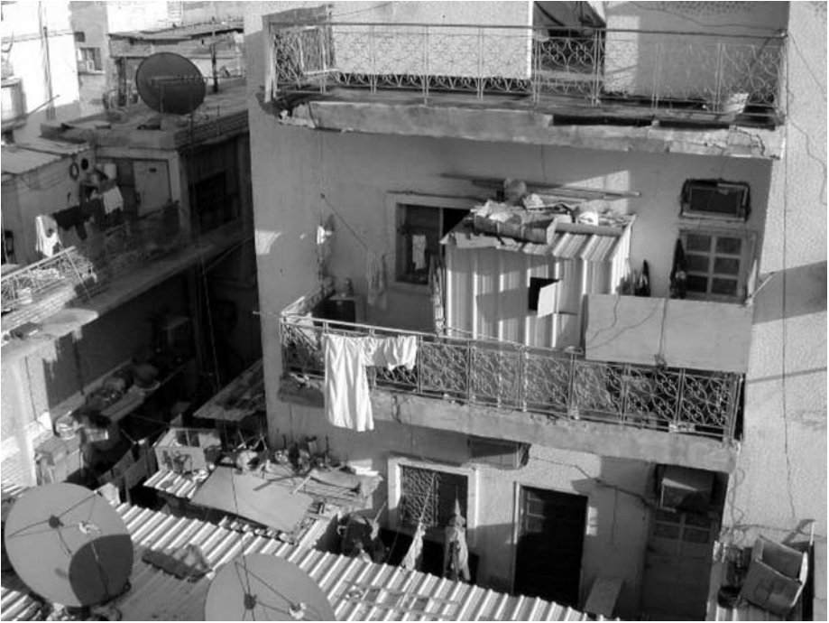
Figure 7.7. Expatriate workers' houses.
