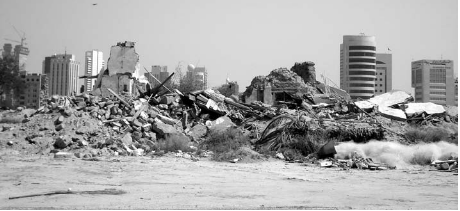
Figure 7.4. Demolished old houses.
