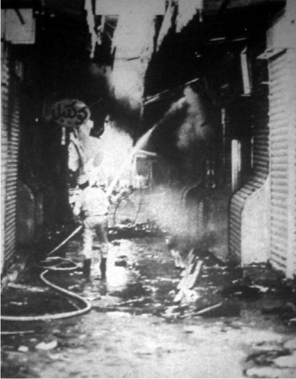
Figure 4.7. Tackling the fires in the souqs , September 1975.
