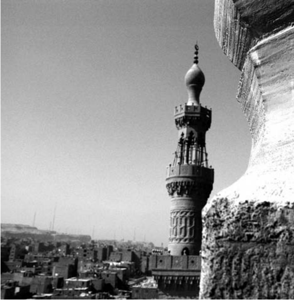
Figure 1.1. The minaret of the Farag ibn Barquq Mosque in Cairo enveloped by informal settlements built in proximity to the City of the Dead.
