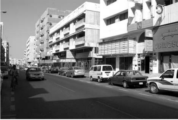
Figure 9.3. The apartment building where I lived with my family between 1978 and 1981.
