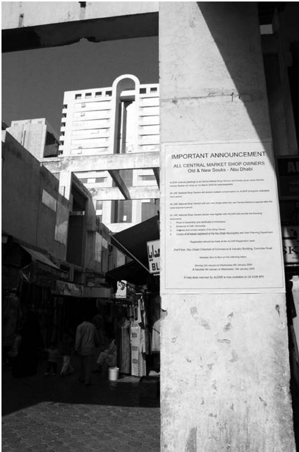
Figure 10.15a. Demolition notices plastered throughout the crumbling complex.
