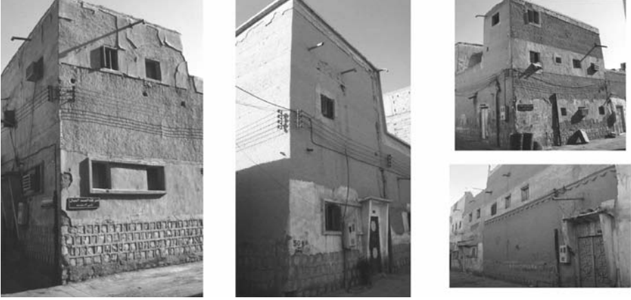
Figure 6.9. The mud surfaces of the traditional houses in Riyadh plastered with cement and the traditional house gate replaced by a concrete one because it reflects modernity.
