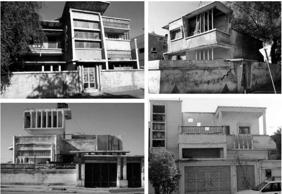
Figure 6.8. A number of villas constructed in the 1950s by the Aramco Home Ownership Program in Dammam.
