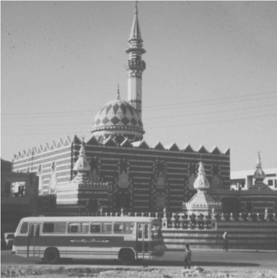
The Ashrafiyyah Mosque in 'Amman uses alternating layers of black basalt and white limestone. This building style is more common in northern Jordan, where both stones are found. Courtesy of the author.
